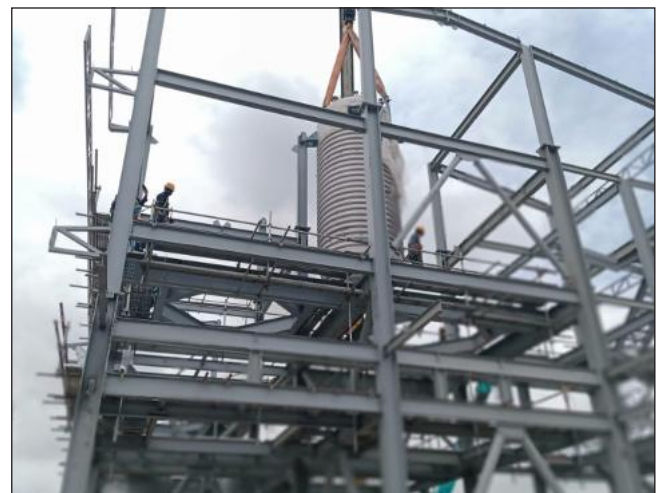
Erection Vessel 20-R-002, Weigh 17 Ton by 100 Ton Mobile Crane
