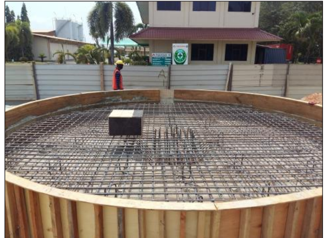
Reinforcement for Tank 100MT
