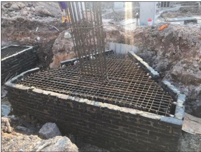
Reinforcement Installation for Foundation Works
