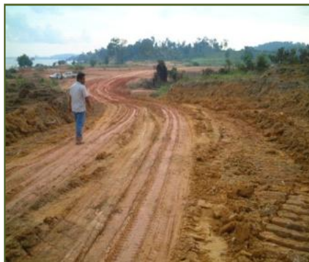
The making of Temporary Access Road
