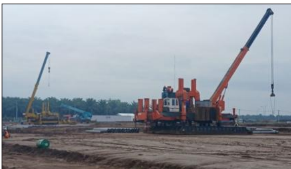
HSPD On Process Piling Work
