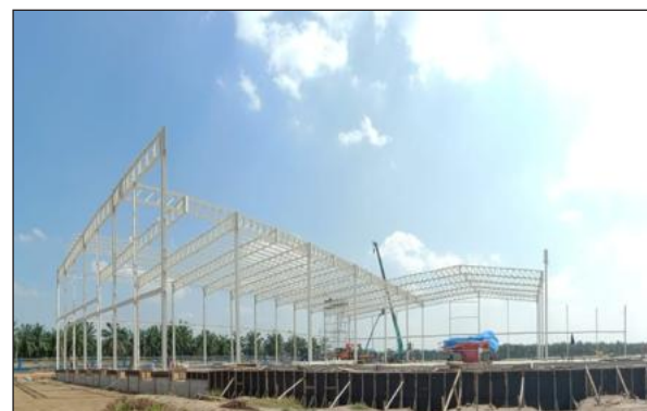
Installing Truss and Tie Beam
