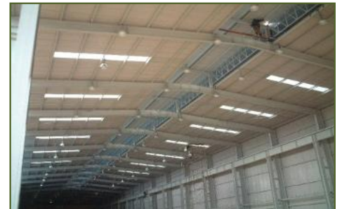
Installation of High Bay Light
