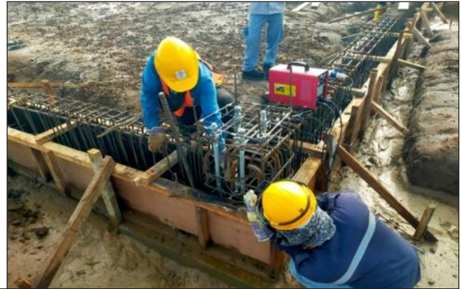
Welding and Installation of Anchor Bolts for Foundations
