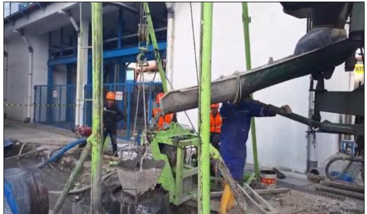
Pouring Concrete Bored Pile
