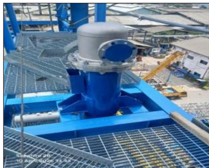
Install Equipment 3E-205 (Condensor) (Elevation +19.000)
