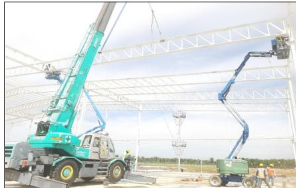
Installing Truss and Tie Beam
