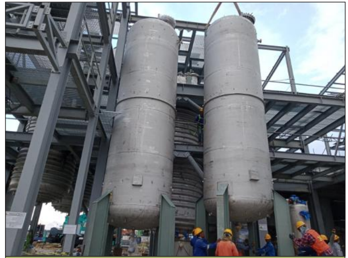
Erection Vessel 20-VE-004B
