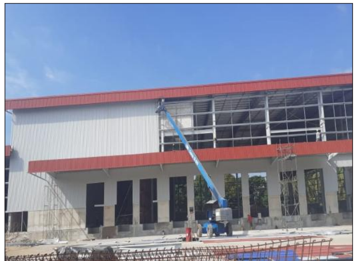
Installation of Wall Cladding
