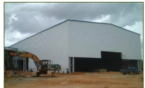
View of Main Building
