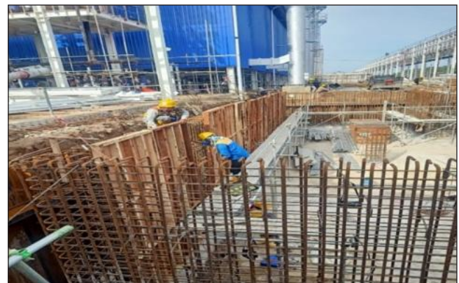
Installation of Retaining Wall Formwork WTP
