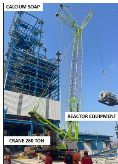
LIFTING OF REACTOR EQUIPMENT
