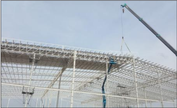
Steel roof truss and purlin installation in progress
