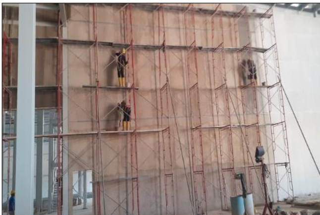
Installation of 12 Meter Brickwall Hight at Raw Material Warehouse Area
