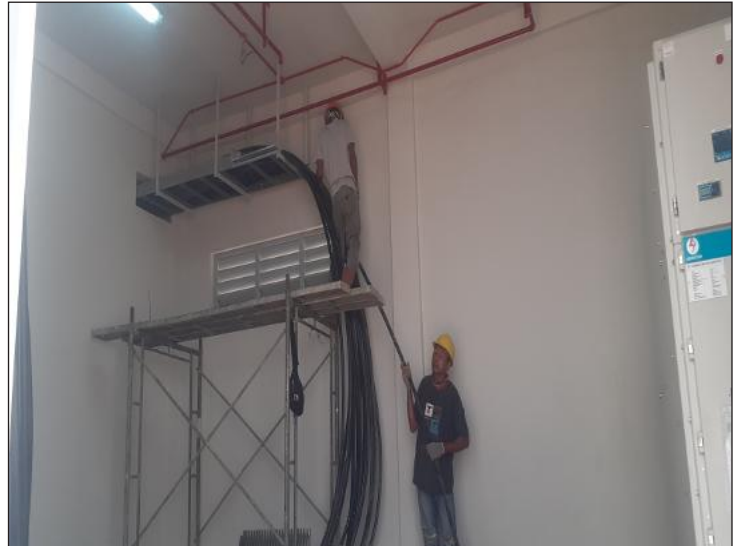
Cable power installation from Substation to MCC Room
