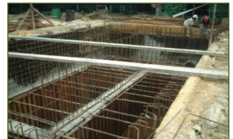
Half of Reservoir Wall Concreted
