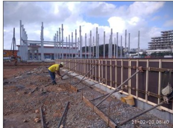
Formwork Installation for Bundwall
