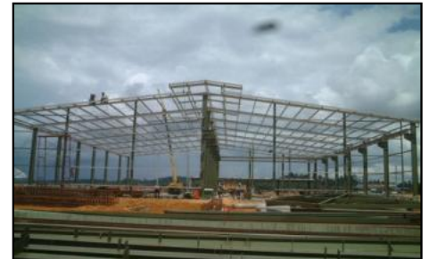
Main Building Steel Structure
