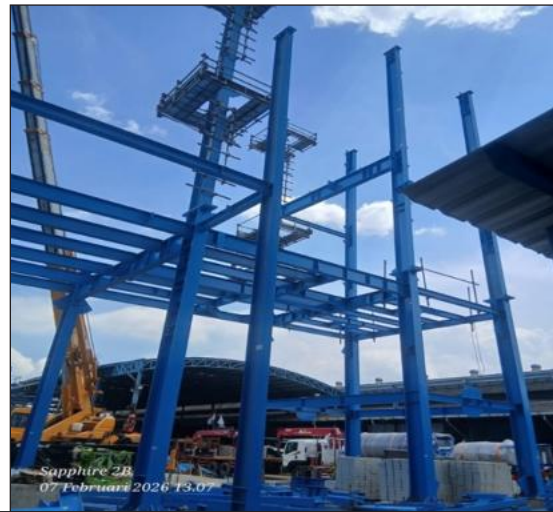
Erection Beam Oil Hydrogenation Plant
