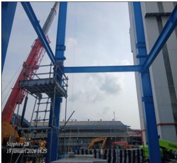
Erection Beam Glycerine & Fatty Acid
