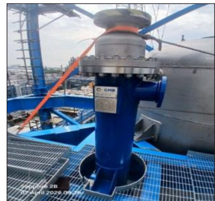
Install Equipment 3C-202 (Vessel Hydrogenation Reactor) (Elevation +19.000)
