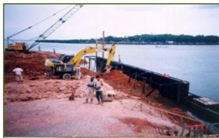
Installation of Steel Structure Wharf
