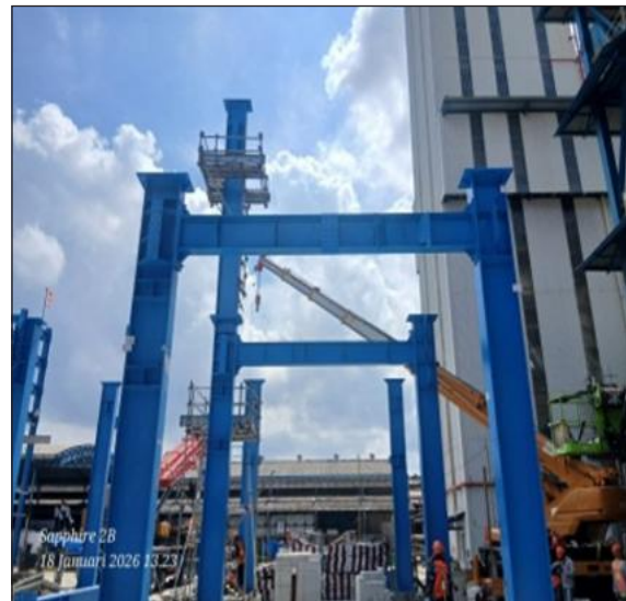
Erection Beam Glycerine & Fatty Acid
