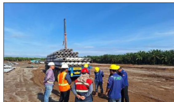
TBM Crew HSPD Before Piling Work
