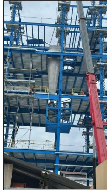
Erection Cyclone Equipment
