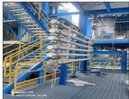
Install Equipment 3E-203 (Heat Recovery Exchanger)(Elevation +7.000)
