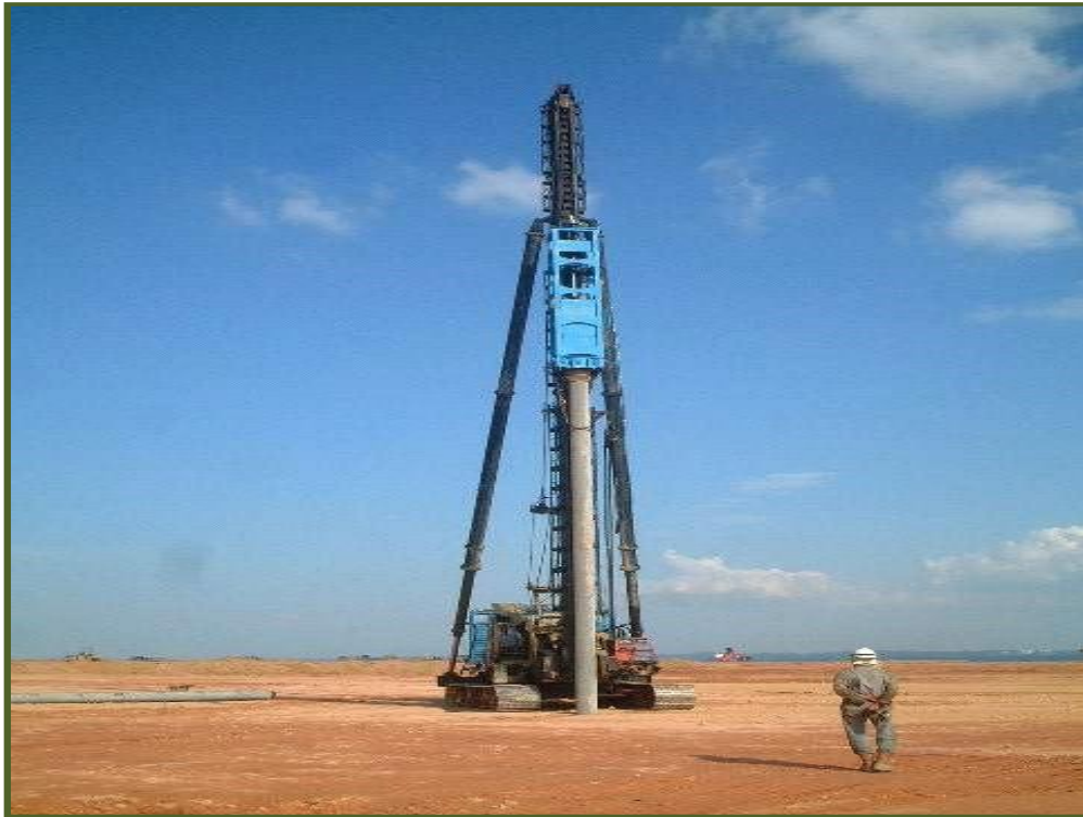
Driving Pile by Hydraulic Pile Machine
