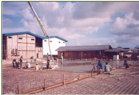
Slab Concreting
