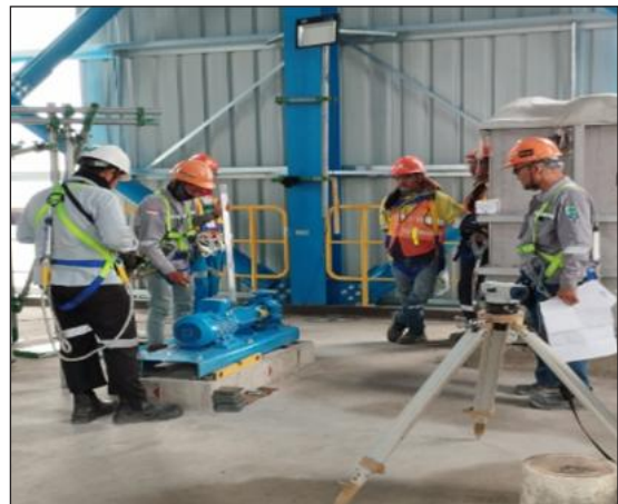
Pump of Levelling and Centerline
