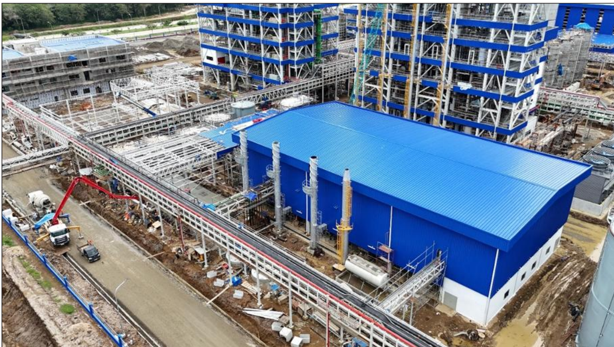
Side view of the boiler house
