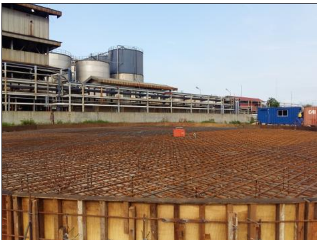
Reinforcement for Tank 3000MT
