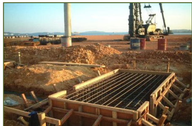
Formwork & Reinforcement for Pile Cap
