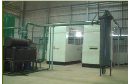
Installation of Factory Equipments
