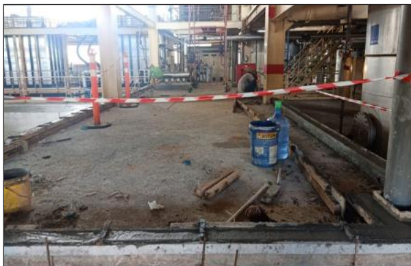
Pouring of Concrete
