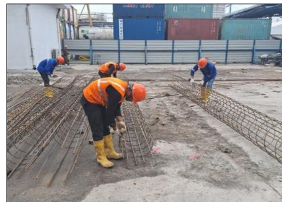
Rebar Bored Pile Fabrication
