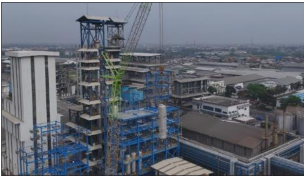
Install Equipment 3C-754 Using Crane 260 Ton (Elevation +18.000)
