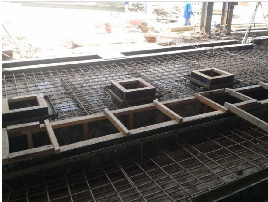
Reinforcement of Waste Water Storage Tank Works
