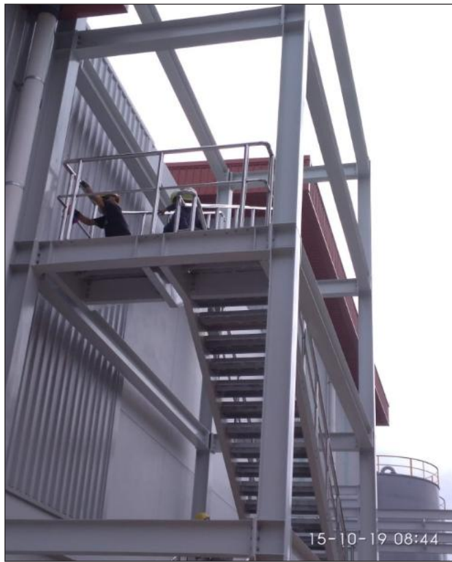
Erection of Staircase for Condensor Area
