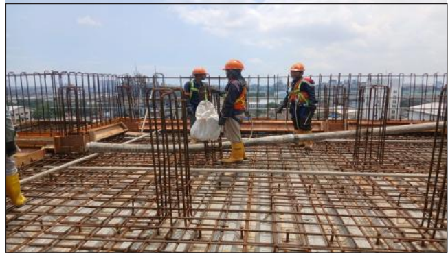
Install Rebar
