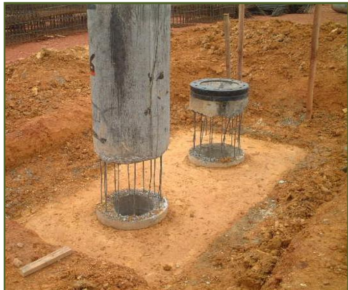
Cut of Pile
