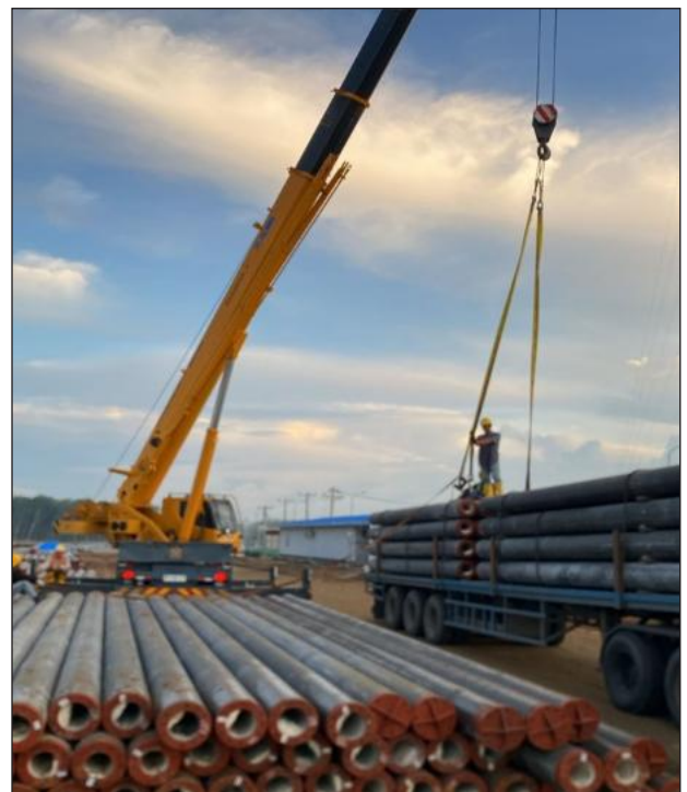
Process Unloading Material Pile By Crane
