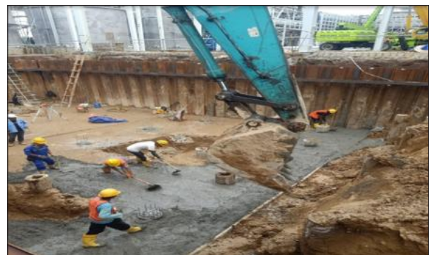
Pouring Concrete Lean Concrete Pile Cap
