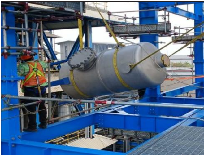
Install Equipment 3D-752 (Saponification Vessel) (Elevation +12.000)
