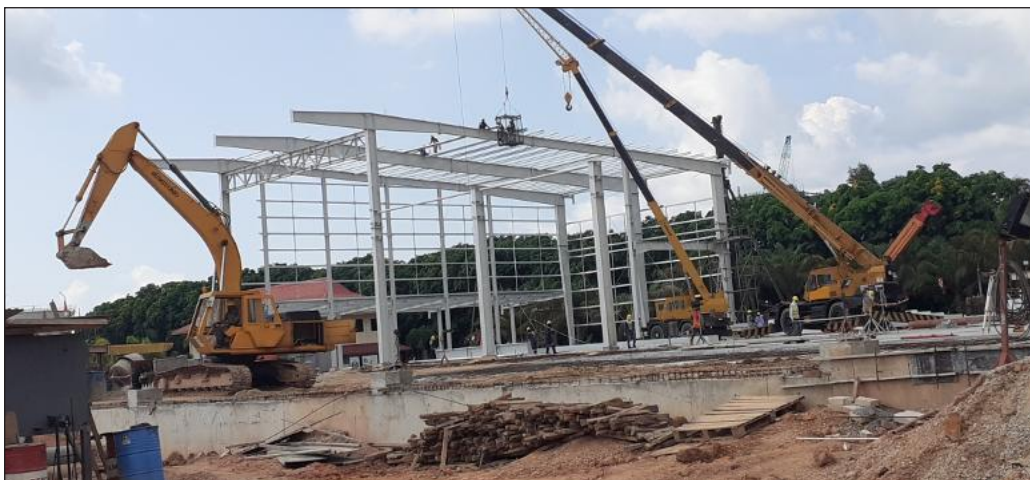
Erection of Roof Purlin
