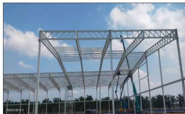
Installing Purlin Roof at Warehouse
