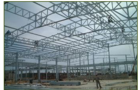
Steel Structure Erection
