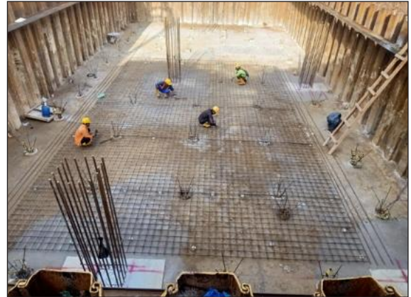
Base Slab Reinforcement Works
