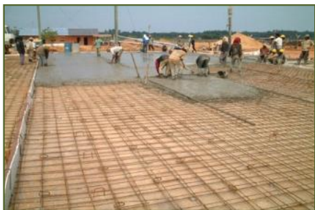
Slab Concreting
