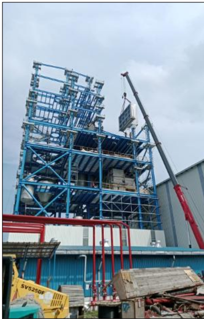
Erection Heat Exchanger
