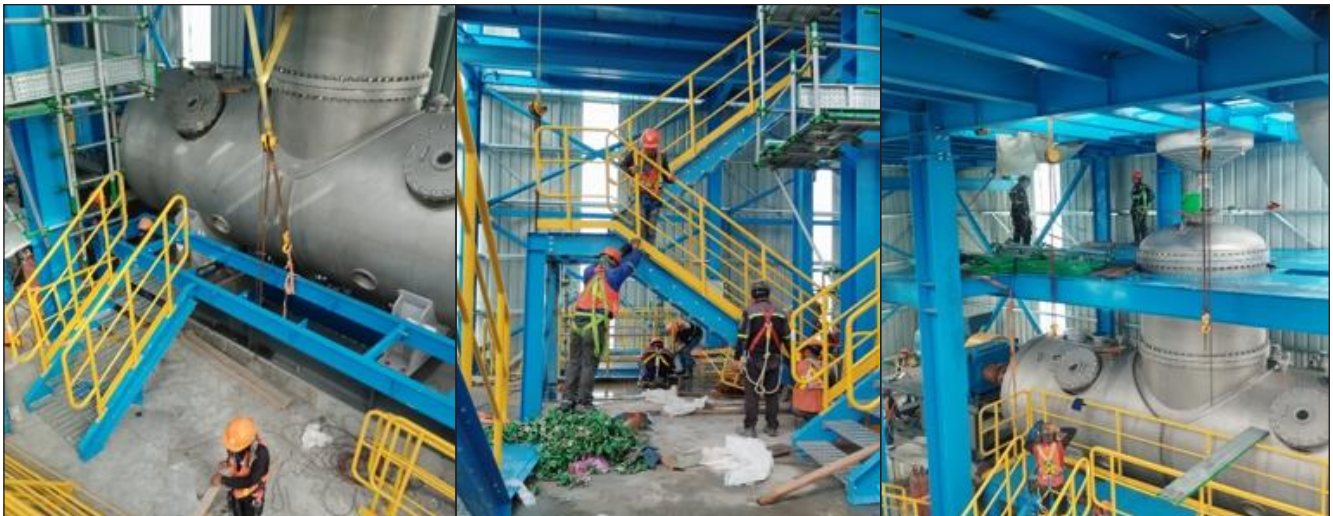
INSTALLATION OF STEEL STRUCTURE COLUMN, BEAM, CHECKER PLATE AND HANDRAIL
