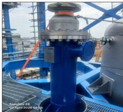
Install Equipment 3C-202 (Vessel Hydrogenation Reactor) (Elevation +19.000)
