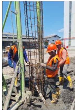
Instal Rebar Bored Pile
