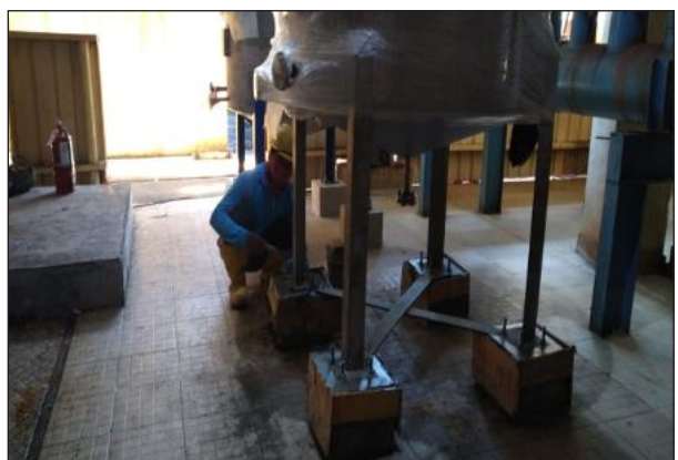
Grouting of Foundation Equipment
