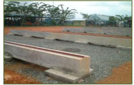
Concrete Base Beam
