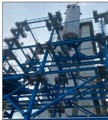
Install Equipment 3C-202 (Vessel Hydrogenation Reactor) (Elevation +19.000)
