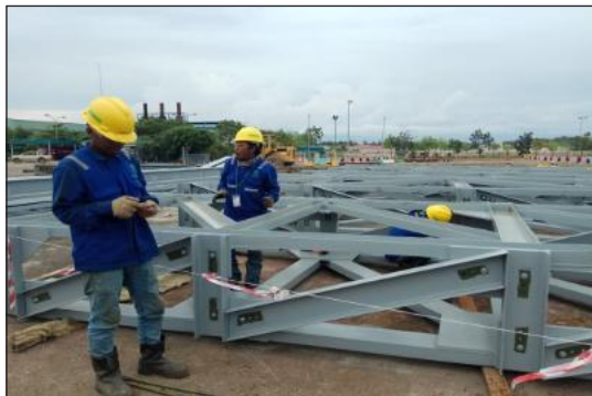
Fabrication of Truss
