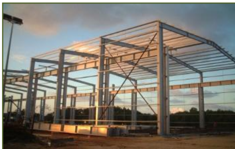
Steel Structure of Main Building
