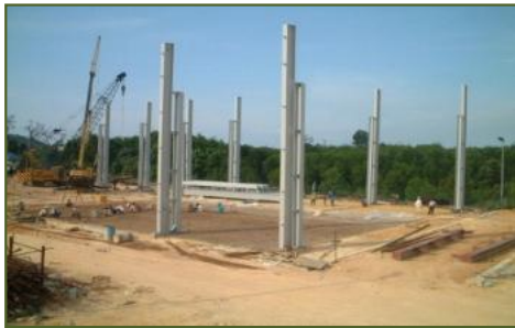
Steel Column Erection
