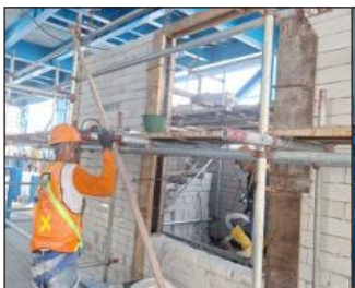
Install Brickwall Marshalling Room
