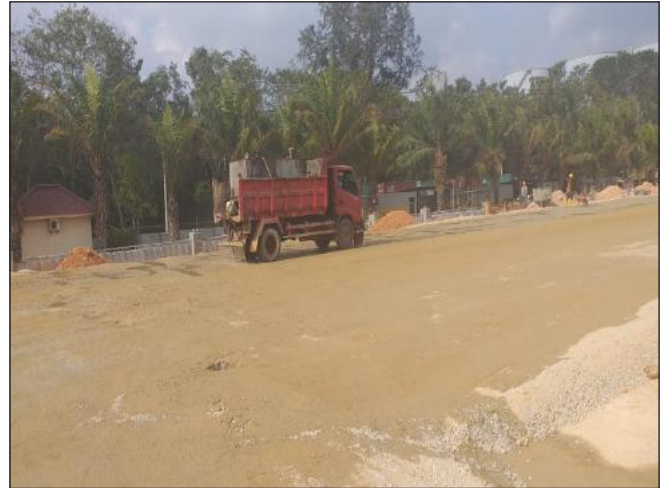
Curing Crusher Run
