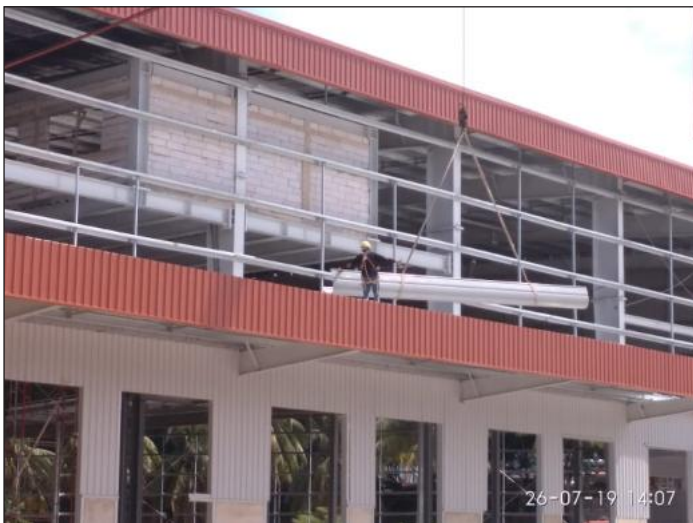
Installation of Wall Cladding
