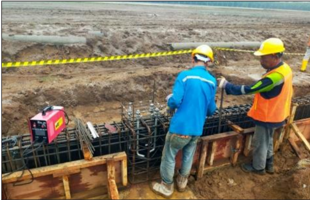
Welding and Installation of Anchor Bolts for Foundations
