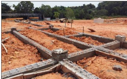
Concrete Structure Works
