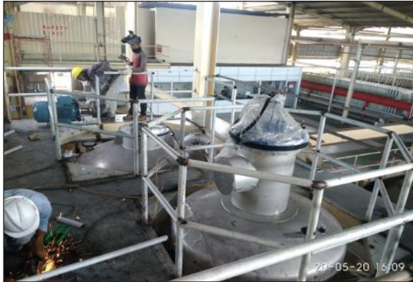
Installation of Railing
