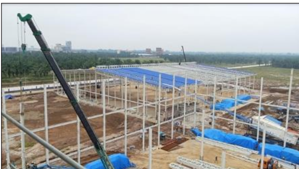
Roof installation using Roll on Site Metal Sheets
