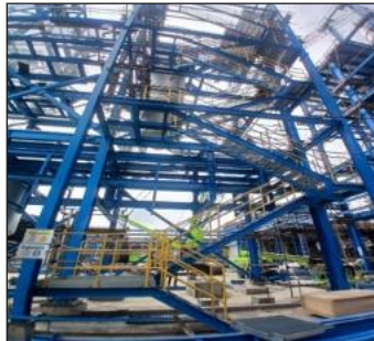
Erection Staircase Oil Hydrogenation Plant
