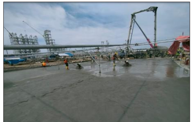
Concrete Floor Leveling and Compaction
