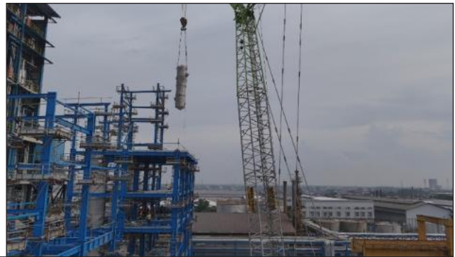
Install Equipment 3C-754 Using Crane 260 Ton (Elevation +18.000)
