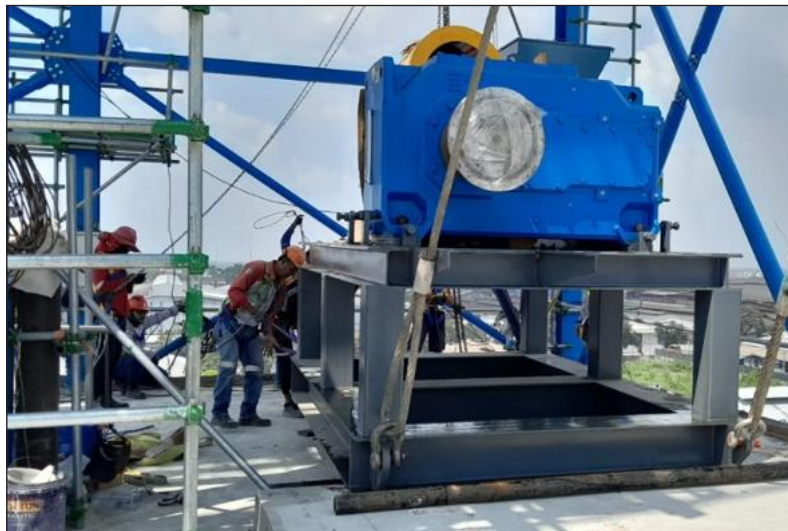
THE MOTOR EQUIPMENT ALREADY ON PLACE
