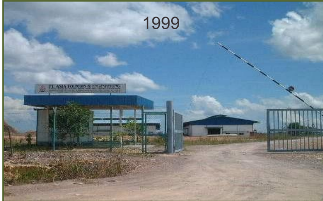
PT. ASIA FOUNDRY ENGINEERING (Factory & Building Renovation)
