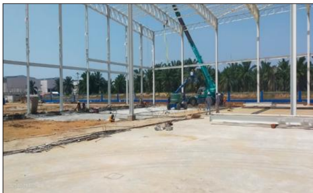
Installing Grider and Truss at Warehouse
