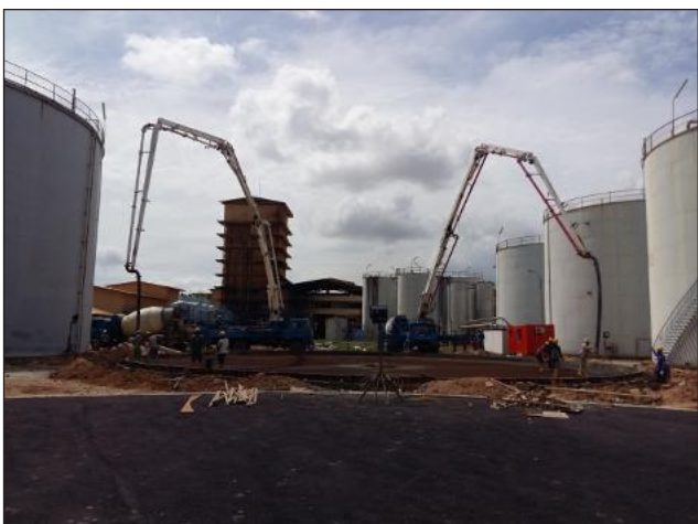
Concreting for Tank 7500MT
