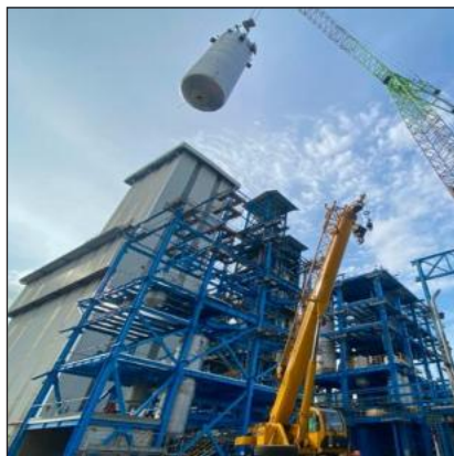
Install Equipment 3C-202 (Vessel Hydrogenation Reactor) (Elevation +19.000)
