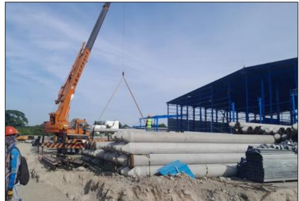
Loading & Unloading Material Pile
