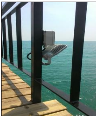
Installation of Lightings
