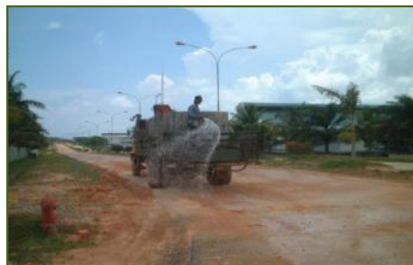
Water Tank Mounted Truck for Road Cleaning & Dust Control
