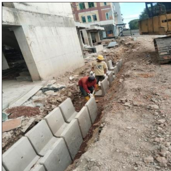
Perimeter Drain Works
