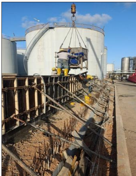
Pouring of Concrete Work
