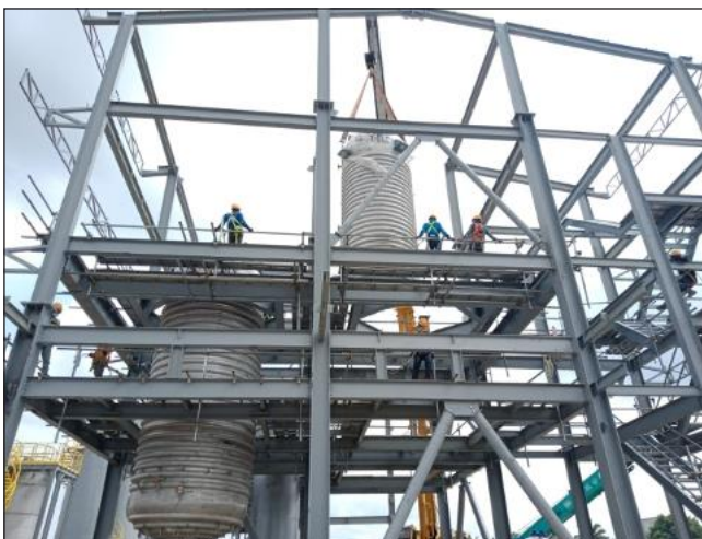
Erection Vessel 20-R-002, Weigh 17 Ton by 100 Ton Mobile Crane
