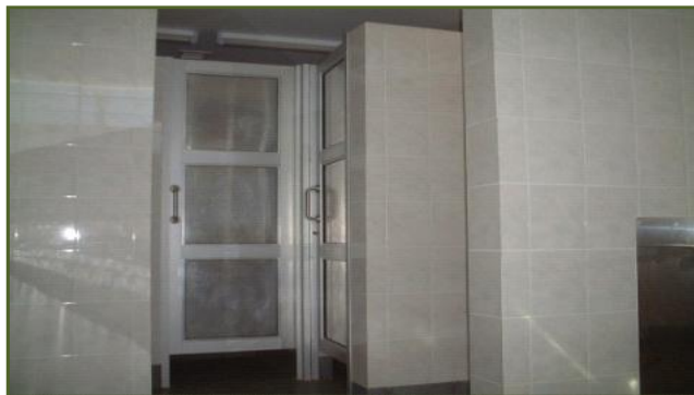
View of Toilet
