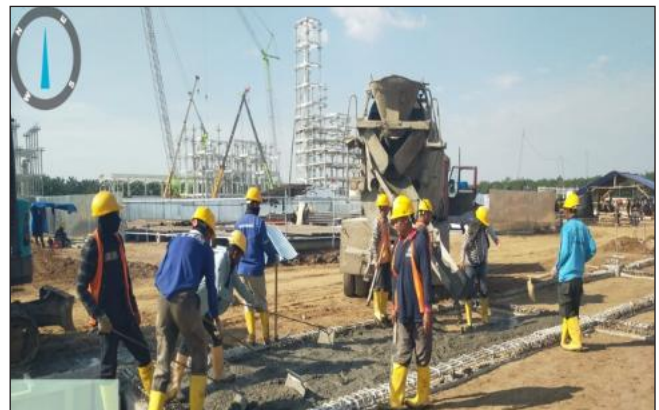
Lean Concrete Works
