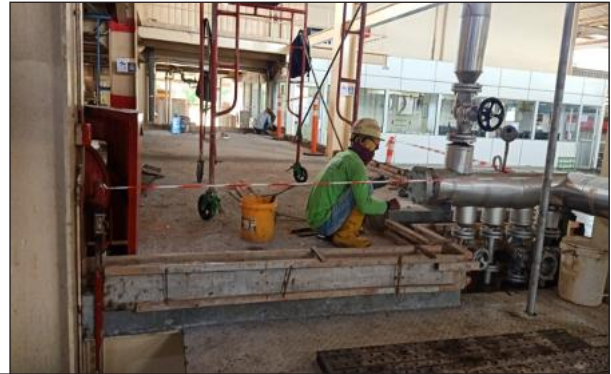
Formwork Installation for Kerb CPO
