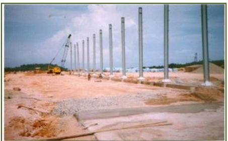
First Erection of Steel Columns
