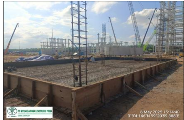
Rebar Panel Installation Area Substation
