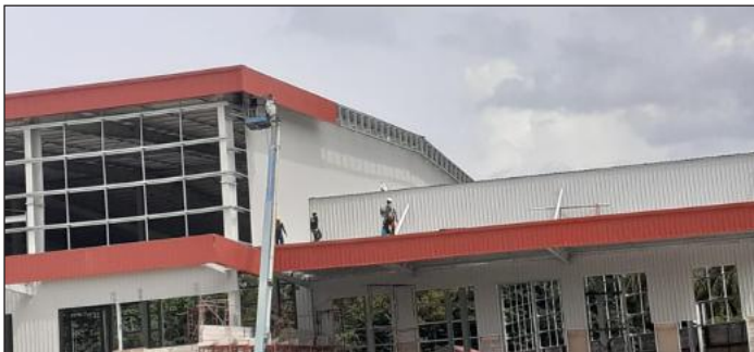
Installation of Facia
