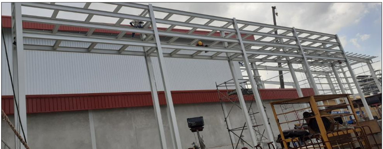
Structure Installation for Pipe Rack
