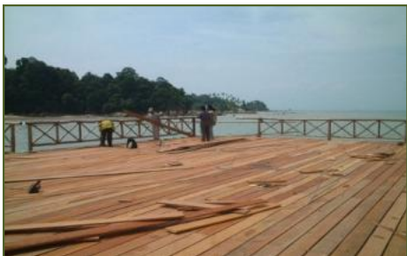
Timber Works at Fishing Deck
