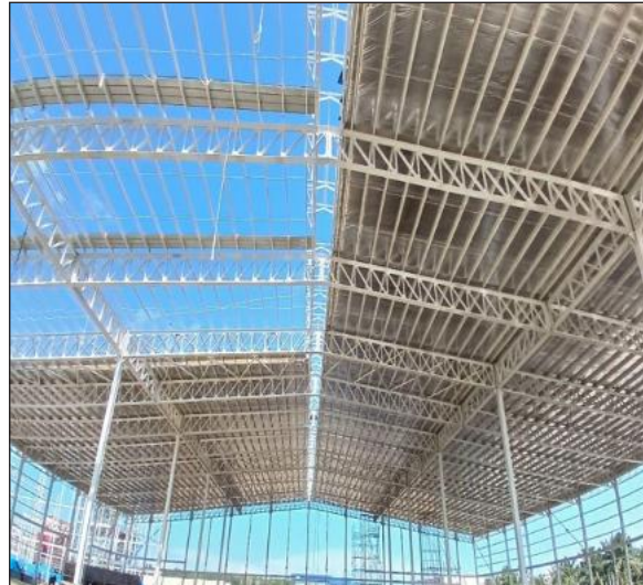
Roof truss installation Warehouse
