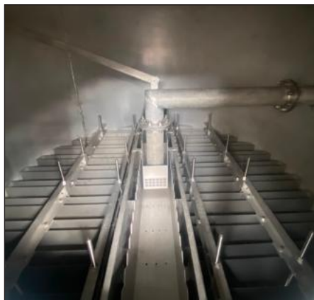
Distributor Installed
