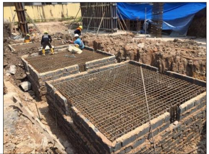
Reinforcement Installation for Foundation Works
