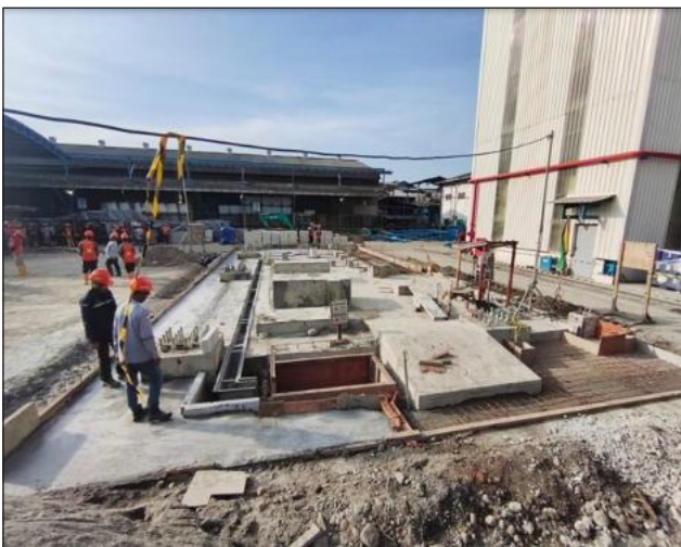
Install Formwork dan Install Lining Fat Trap
