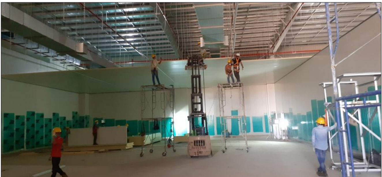
Installation of PIR Panels at Filling Lines Area
