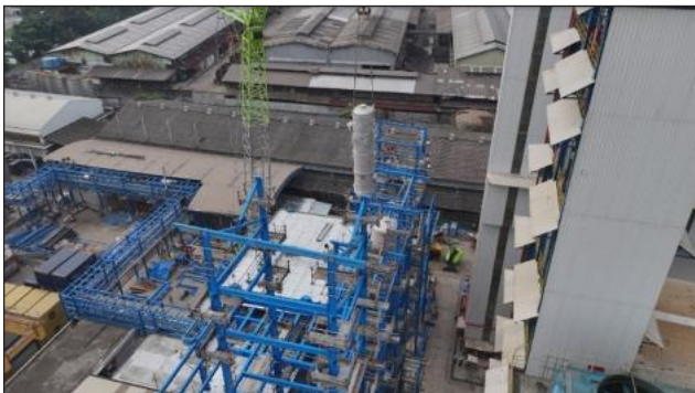
Install Equipment 3C-754 Using Crane 260 Ton (Elevation +18.000)
