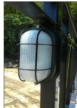
Installation of Lightings
