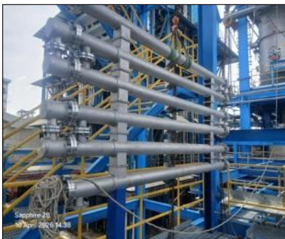
Install Equipment 3E-203 (Heat Recovery Exchanger)(Elevation +7.000)
