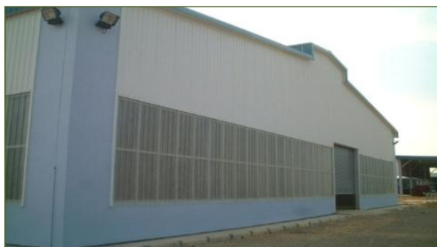
Trancluent Fibreglass for Wall Clading
