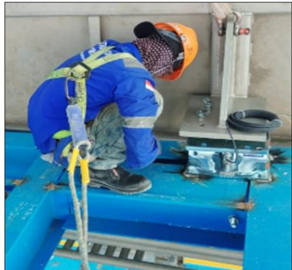
Install Lotsheel Tank D-661 Setting Tank D-661
