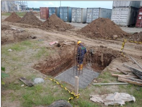
Pipe Rack Foundation
