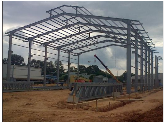
Steel Structure Works
