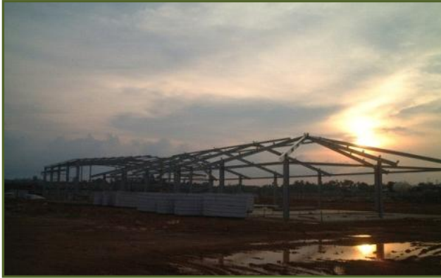
Steel Structure Frames of Content & Prayer Rooms - Warehouse
