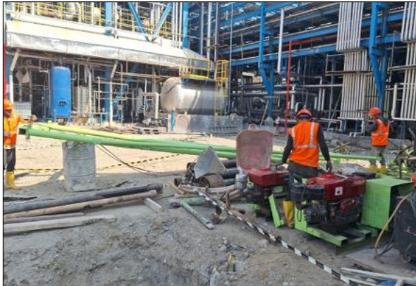
Assembling Equipment Bored Pile
