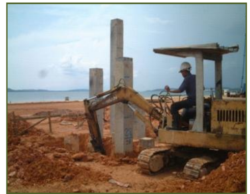
Excavation of Earth
