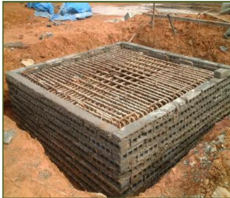
Reinforcement & Formwork for Foundation
