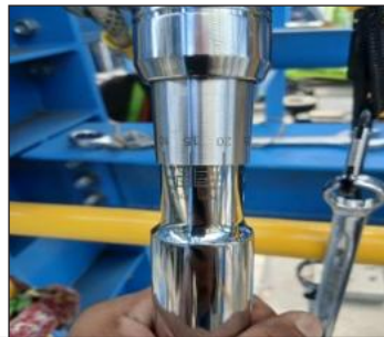
Torque Tightening Bolt
