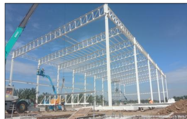
Installing Truss and Purlin
