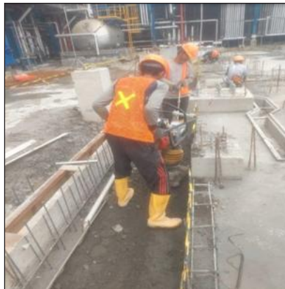
Rebar Installation and Foundation Concrete Casting with Proper Compaction
