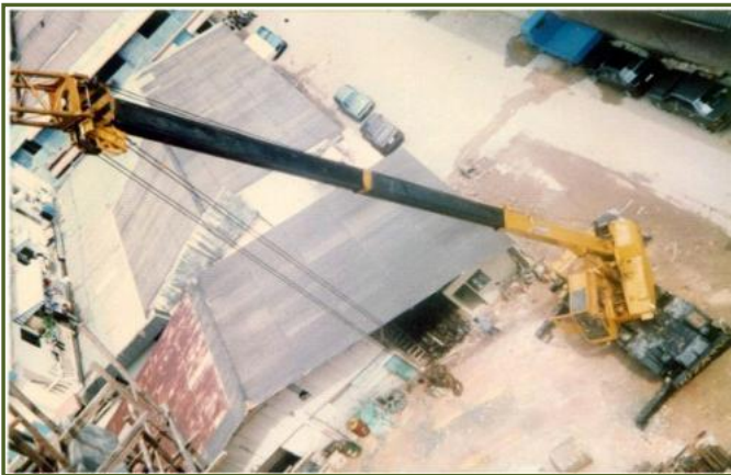
Use of Mobile Crane for High Rise Building
