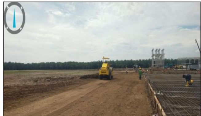
Soil Compaction and Leveling
