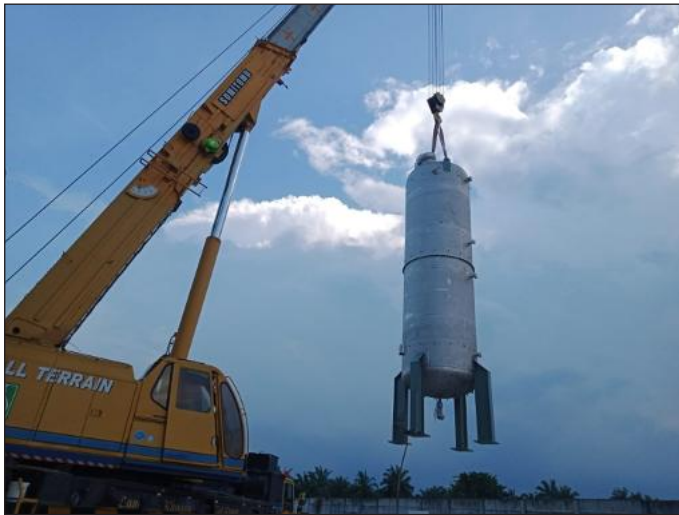
Erection Vessel 20-VE-004A
