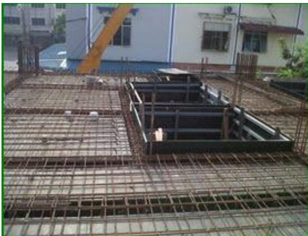
Floor Slab Works
