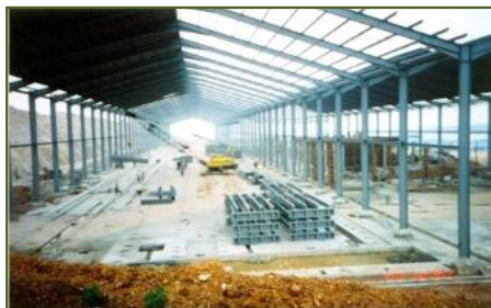
252 M Long x 52 M Wide Steel Structure
