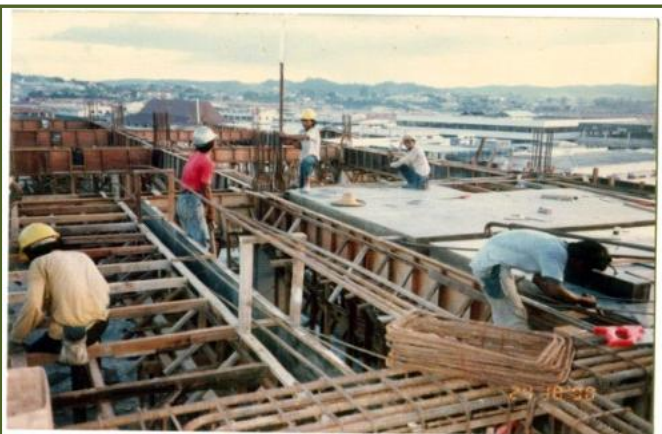
Formwork for Level 4
