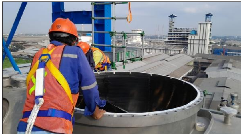
GASKET INSTALLATION
