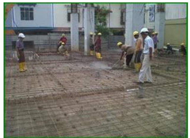
Concrete Slab Works
