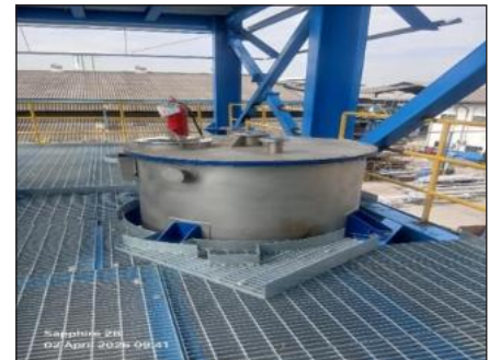
Install Equipment 3D - 201 (Deareator Heater) (Elevation +7.000)
