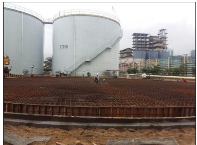
Reinforcement for Tank 7500MT
