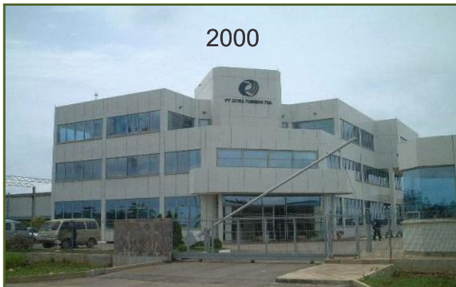
PT. CITRA TUBINDO Tbk. (Headquarter's Office Renovation Electrical Works)
