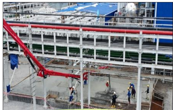
Concrete pouring work using a concrete pump
