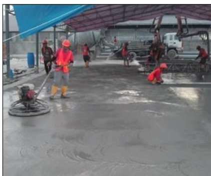
Superflat FF 35 (Tolerance 5 mm/3 m)
