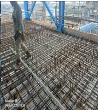
Install Rebar Marshalling Room
