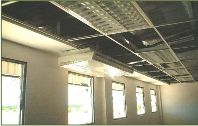
Installation of Aircon
