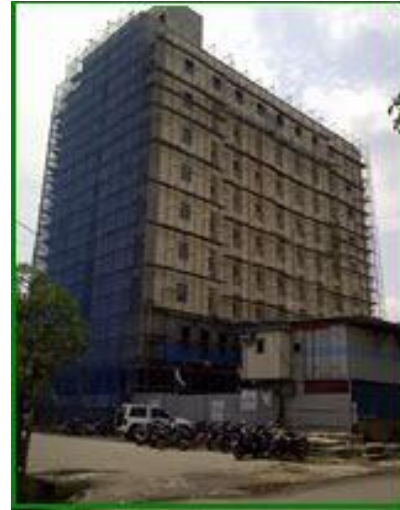
External Wall Works
