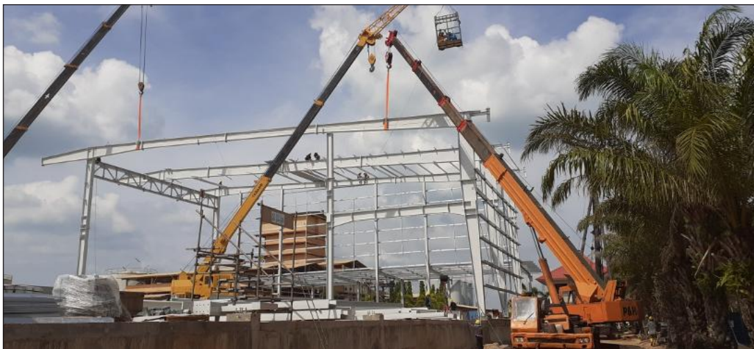
Erection of Rafter
