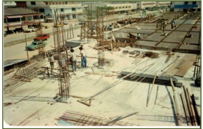
View of Level 2 Formwork in Progress
