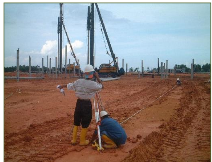
Piling Points Surveying
