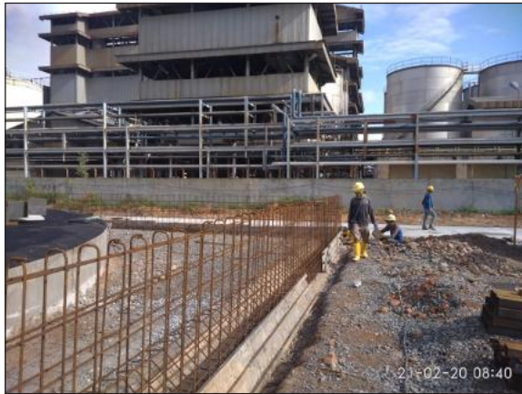
Reinforcement Installation for Bundwall
