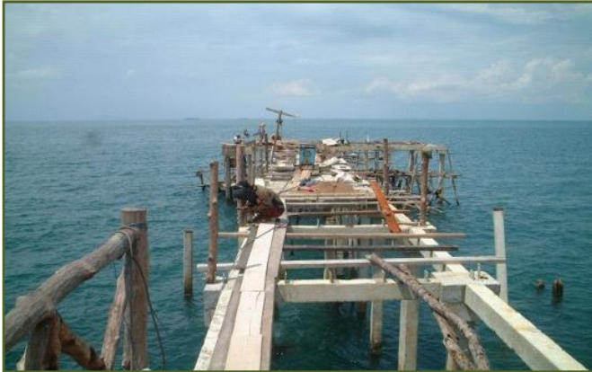
Concrete Structure for Jetty
