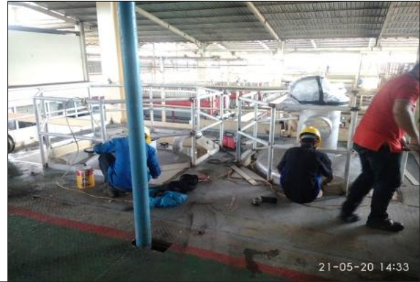
Installation of Railing
