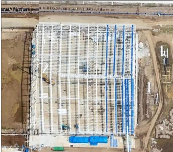
Roof truss installation Warehouse
