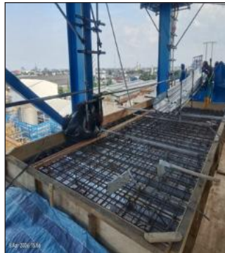
Pouring Concrete Slab Marshalling Room
