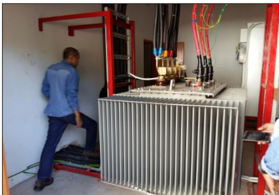
Installation of Transformer
