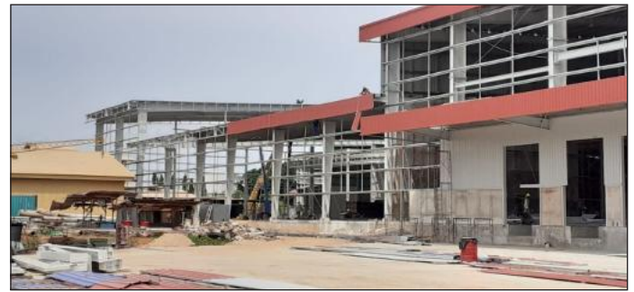
Installation of Facia
