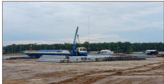
Moving Material Pile To HSPD
