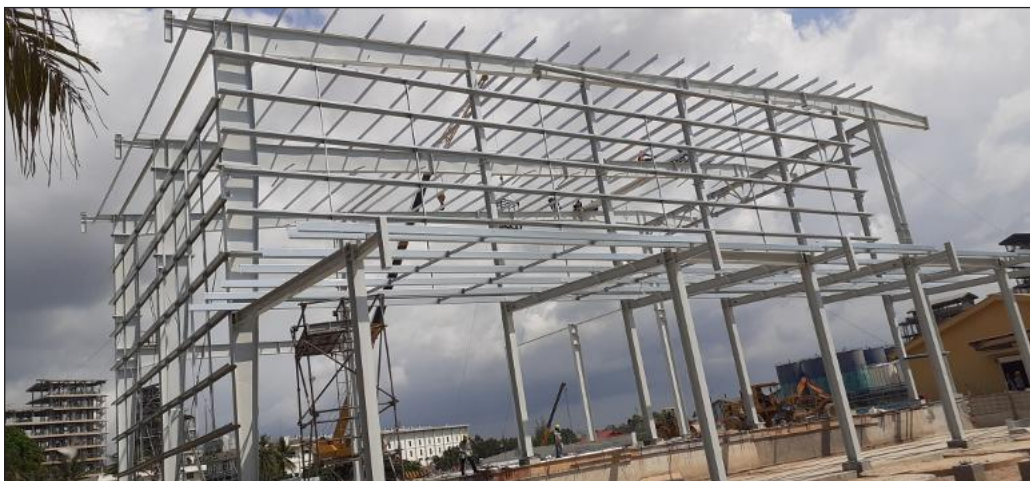
Erection of Roof Purlin
