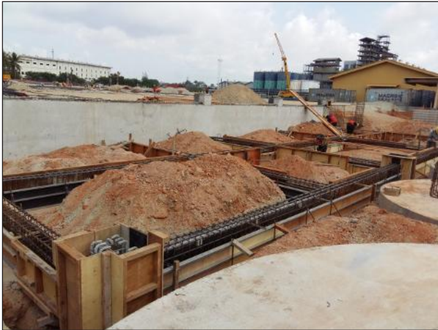
Reinforcement for Ground Beam
