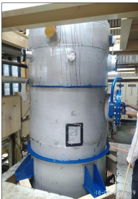
Installation of Oil Vacuum Dryer & Mixing Condenser
