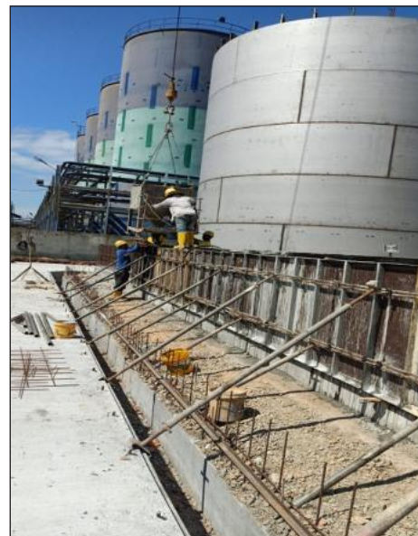
Formwork Installation for Bundwall
