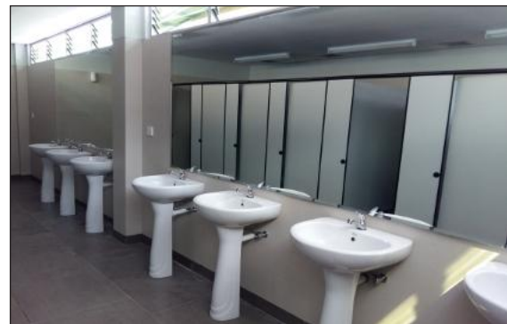
Installation of Wash Basin
