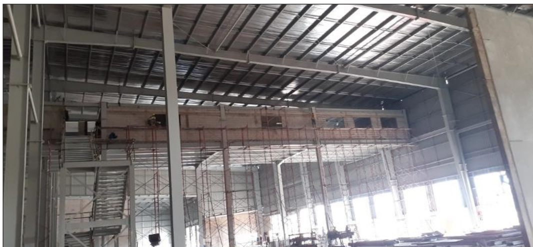
Installation of Brickwall at Mezzanine
