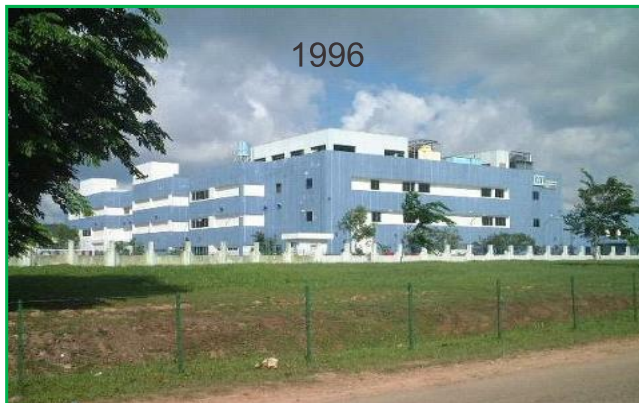
PT. ASTRA MICROTRONICS TECHNOLOGY (Office Renovation)
