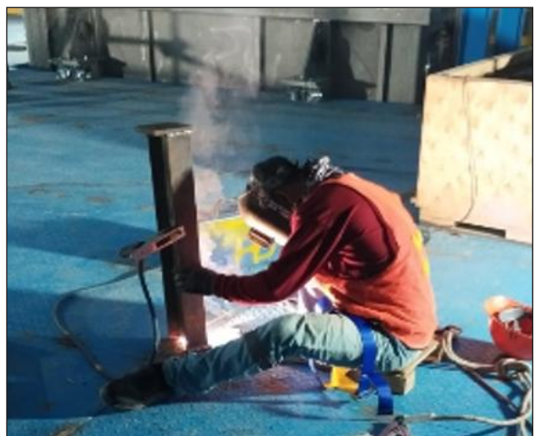
Skid Fabrication D-667
