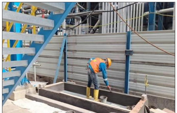
Finishing Bundwall Fat Trap
