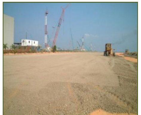
Dust stone/Base Course Finish Level
