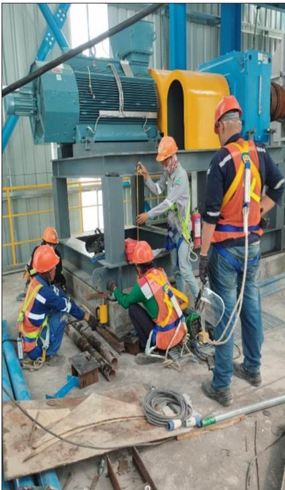
ADJUST POSITION AND ELEVATION OF EQUIPMENT
