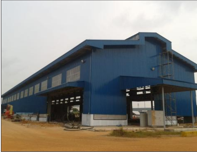
Installation of Roof & Wall Clading
