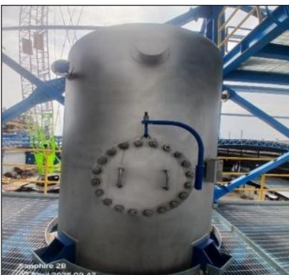
Install Equipment 3D - 203 (Filtered Product Receiver) (Elevation +7.000)
