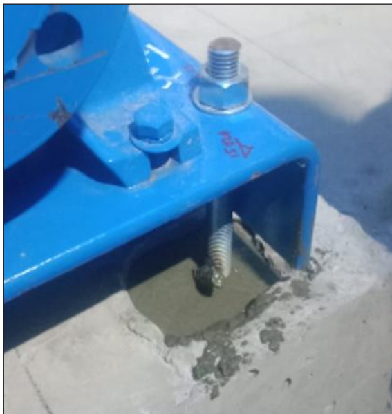
Pump Grouting
