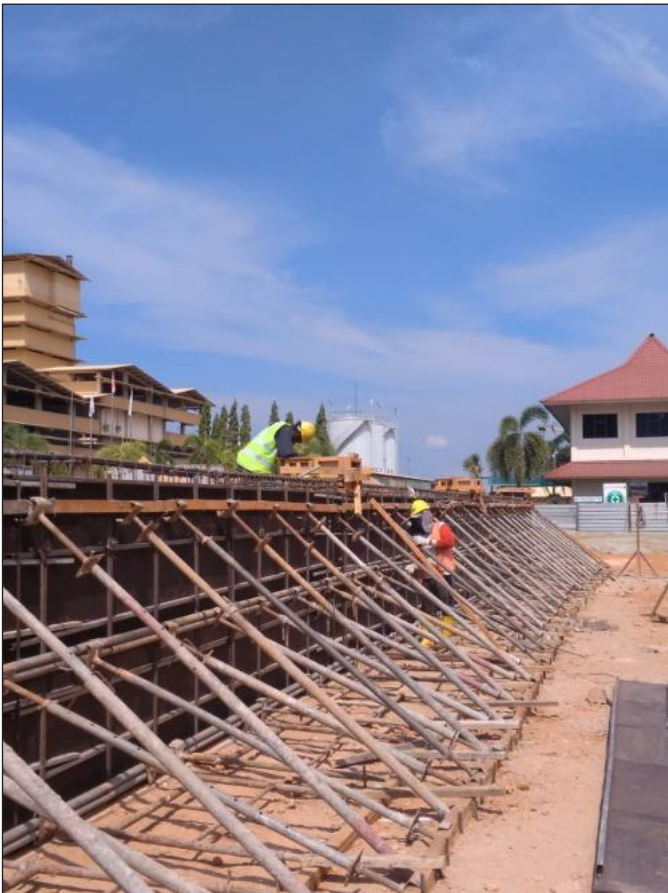
Formwork Installation for Bundwall
