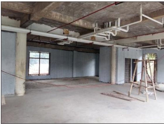
Installation of Plumbing
