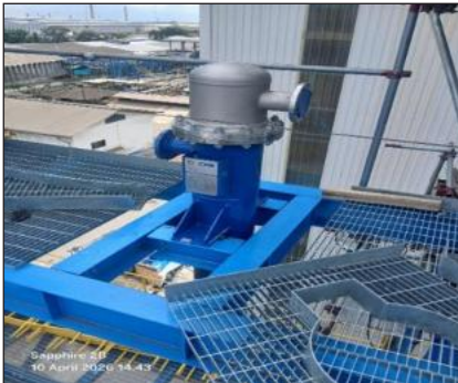
Install Equipment 3E-205 (Condensor) (Elevation +19.000)
