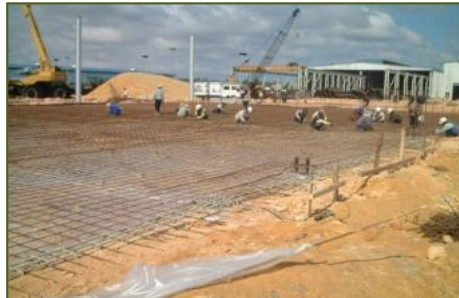
Slab Bar Laying
