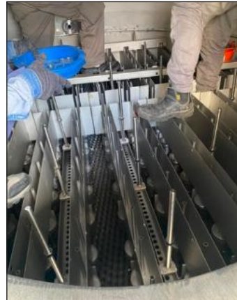
Distributor Installed
