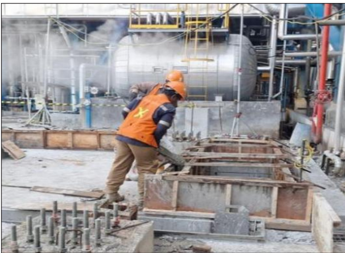
Pouring Concrete Fat Trap
