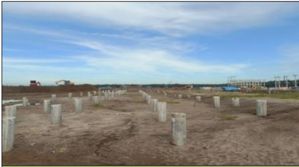
Area Loading Unloading Completed Piling
