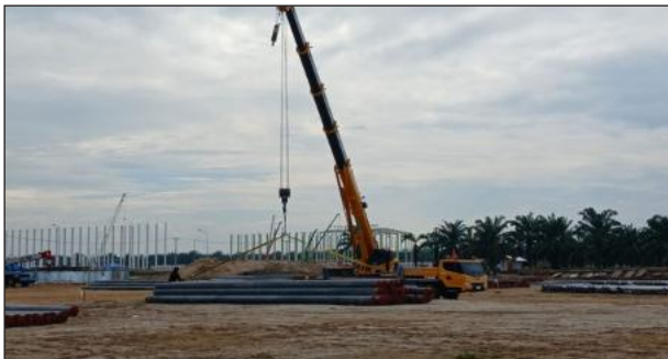
Crane Unloading Material Pile At Laydown
