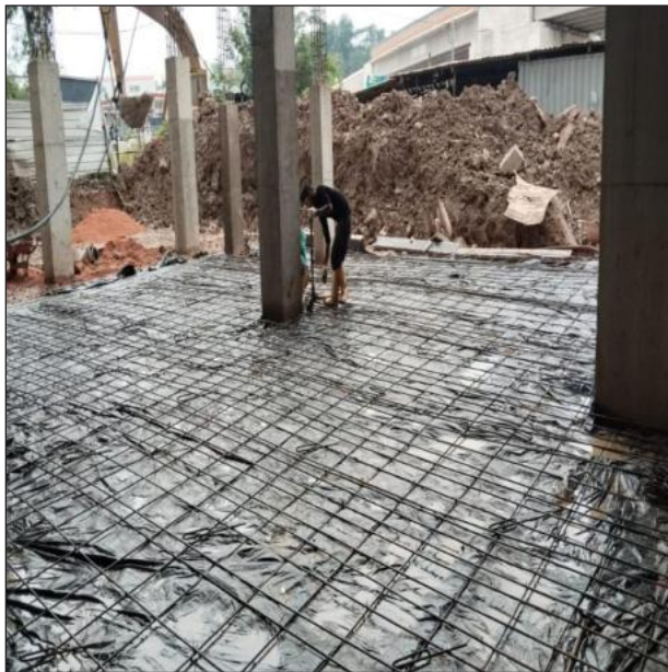
Reinforcement Installation for Slab Works
