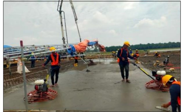
Concrete Compaction in The Warehouse
