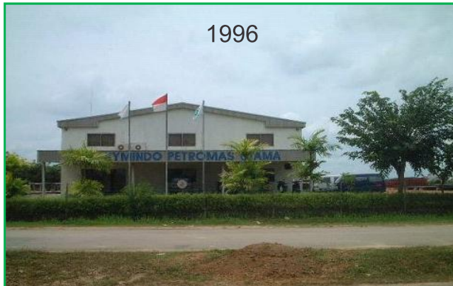
PT. HYMINDO PETROMAS UTAMA (Factory & Yard Repaire)
