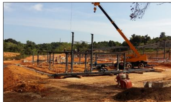
Steel Structure Works
