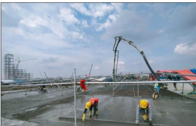
Floor Casting Panel Warehouse
