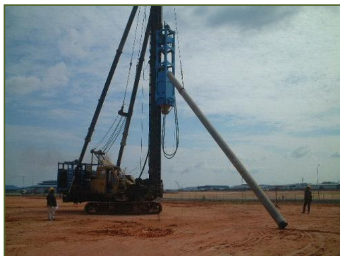
Piling Lifting
