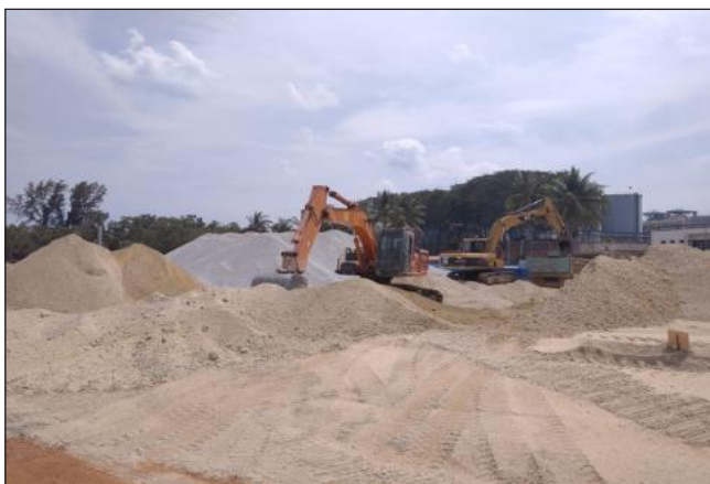
Crusher Run Mixing
