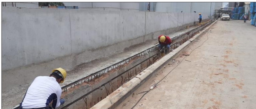
After of Pouring Concrete Work
