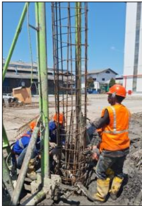
Instal Rebar Bored Pile
