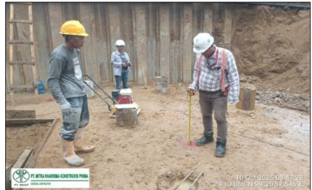
Inspection and Measurement of Ground Level After Compaction
