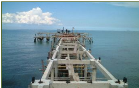
Concrete Pile & Beam
