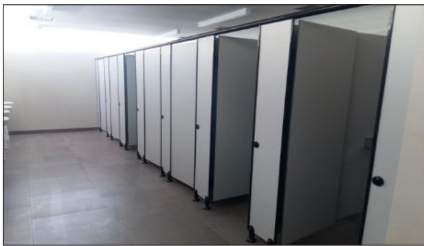
Installation of Cubicle
