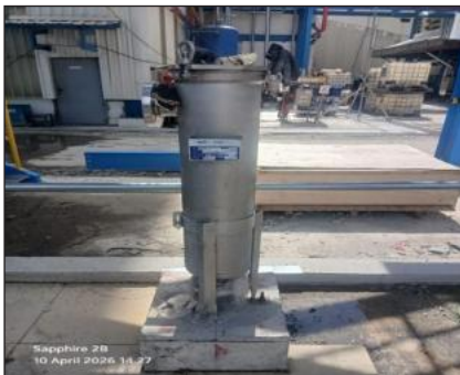
Install Equipment 3F-201B (Feed Filter)(Elevation. 0.000)
