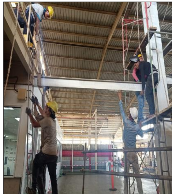
Erection of Steel Beam
