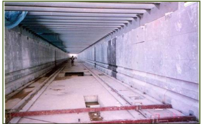
Installation of Prefab Kiln Wall & Roof
