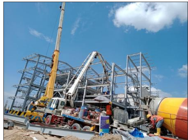
Floor Concreting at Level +5.00 Using Concrete Pump
