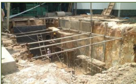
Steel Piling & Concrete Formwork for Reservoir Wall
