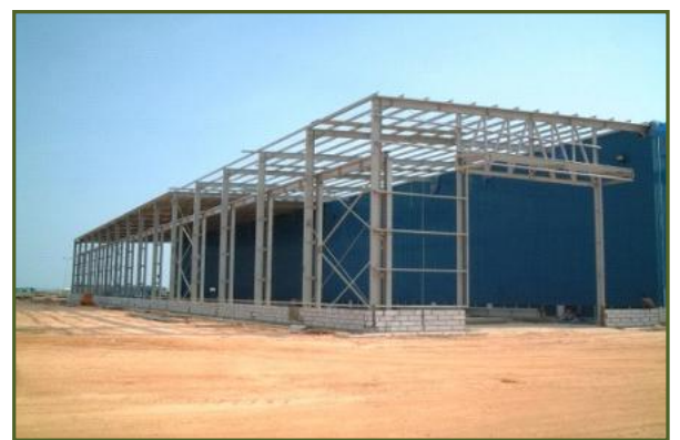
Steel Structure Frames of Pipe Shop
