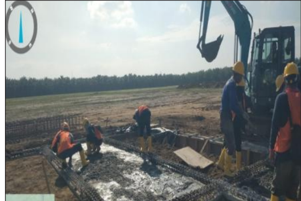
Execution Of Lean Concrete Work At Apron Area
