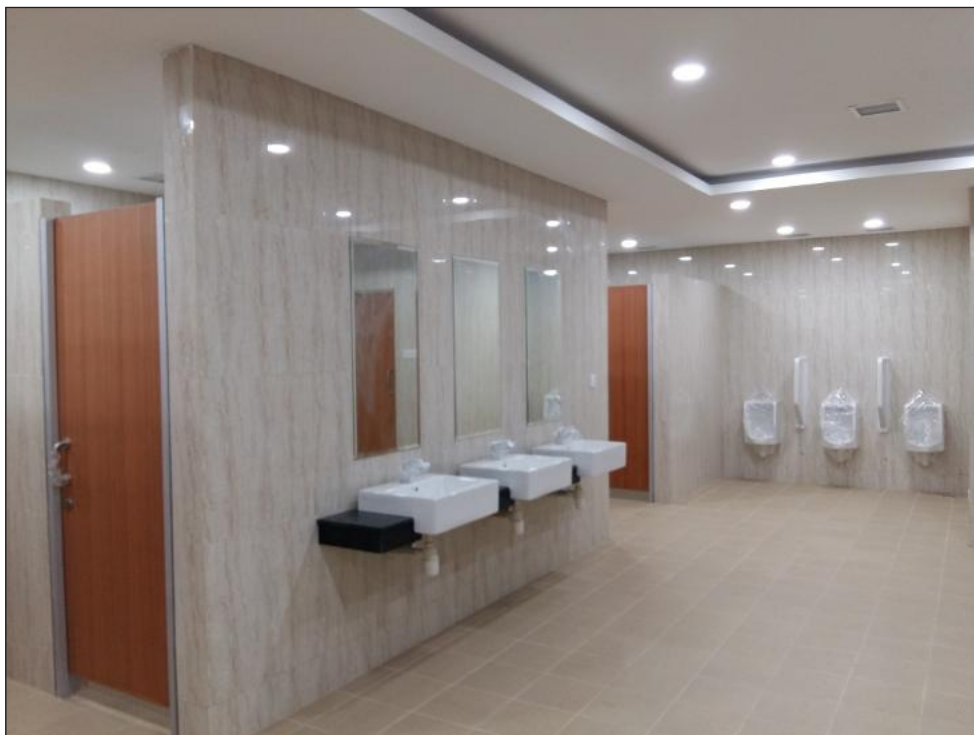
Sanitary Wares and Ceramics Work at Male Toilet
