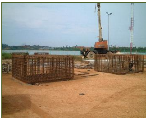
Reinforcement for Foundation
