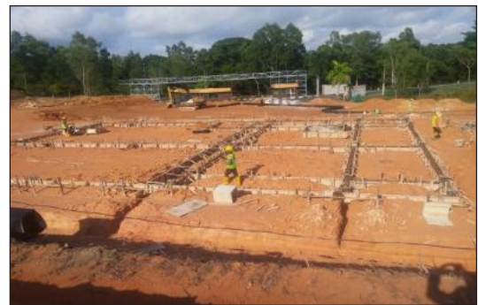
Installation of Formworks
