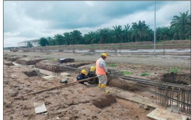
Rebar Installation
