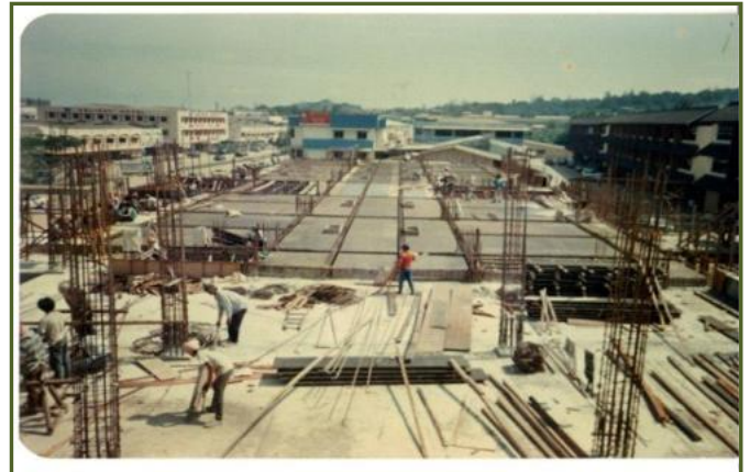
View of Level 2 Partial Concreting
