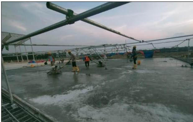
Concrete Floor Finishing Process
