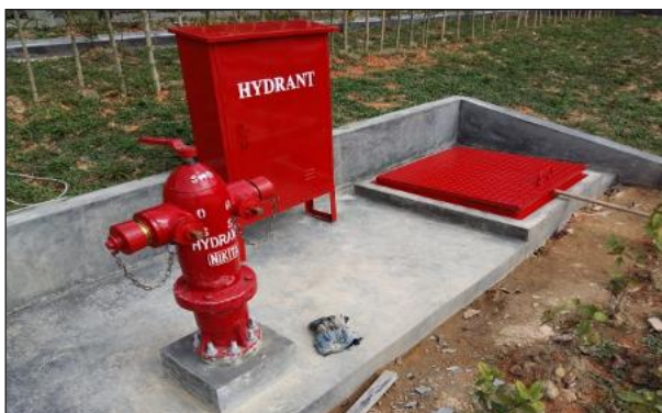
Installation of Hydrant
