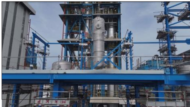
Install Equipment 3C-754 Using Crane 260 Ton (Elevation +18.000)
