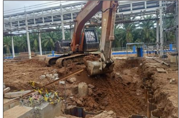
Sheet Cap Excavation
