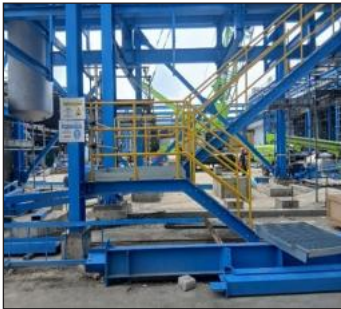
Erection Staircase Oil Hydrogenation Plant
