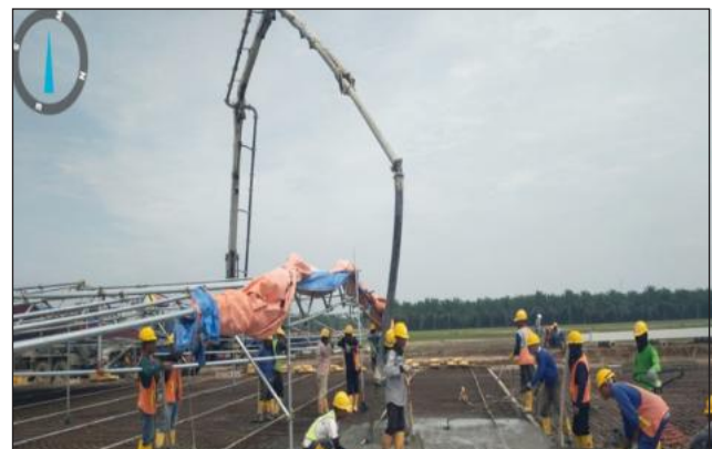
Floor Casting Panel Warehouse
