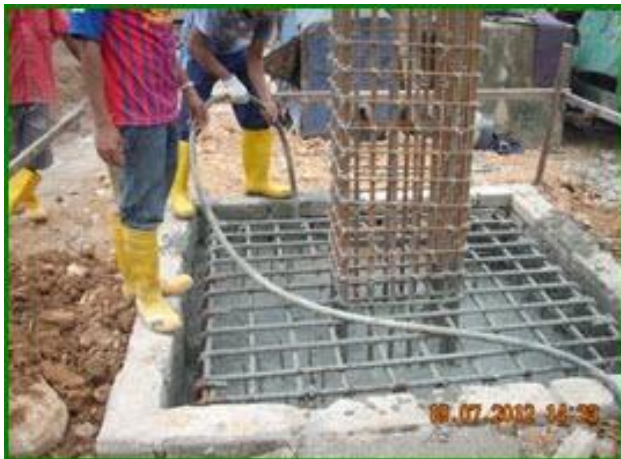
Pile Cap Works
