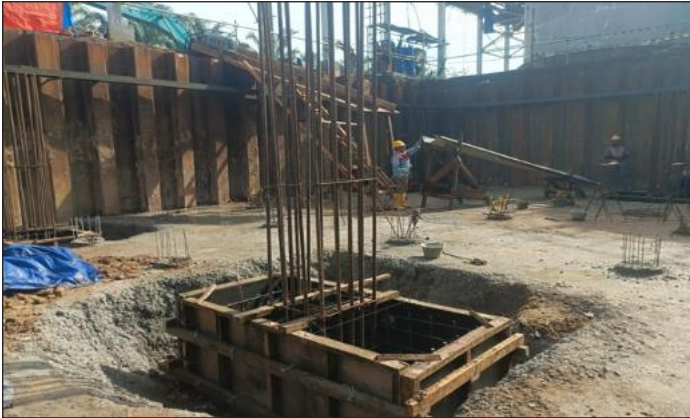
Rebar Installation and Formwork for Column
