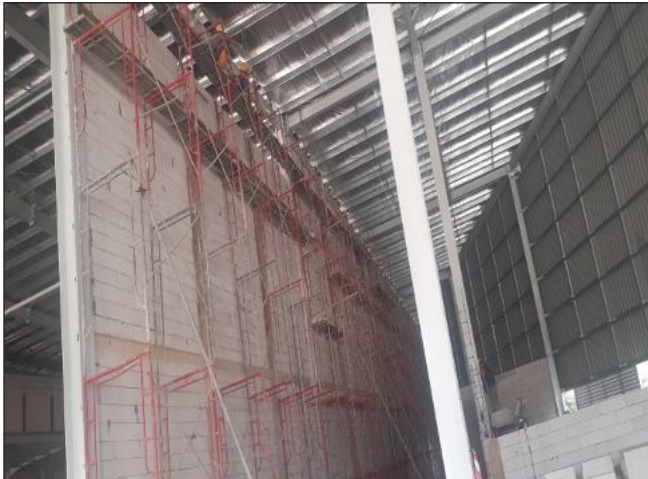
Installation of 12 Meter Brickwall Hight at Finish Good Warehouse Area
