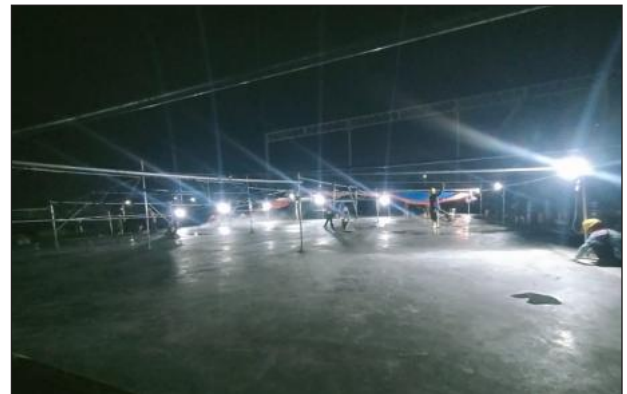
Concrete Floor Finishing Process
