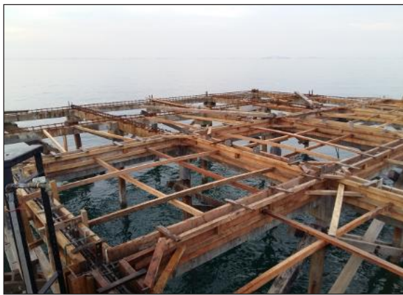
Installation of Formworks
