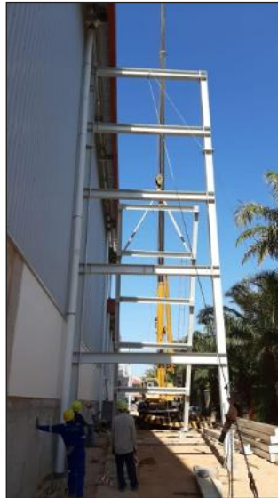
Erection of External Staircase for Mezzanine
