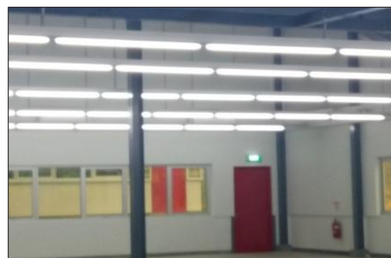
Installation of Lighting
