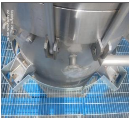
Install Equipment 3F - 202A (Catalyst Filter)(Elevation +13.000)
