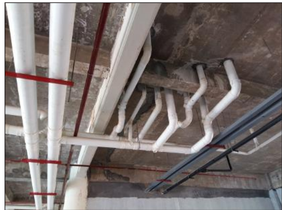
Installation of Plumbing
