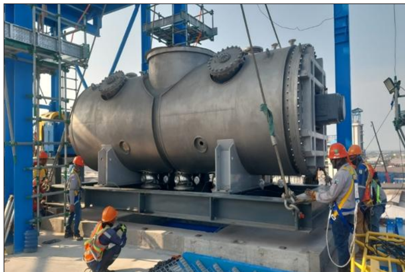
THE REACTOR EQUIPMENT ALREADY ON PLACE
