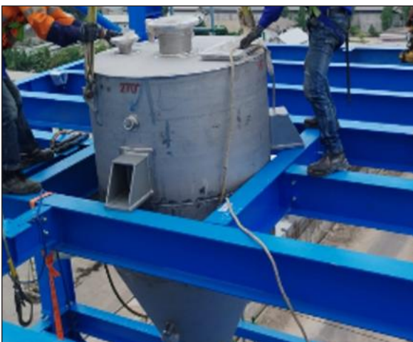
Tank Lifting D-667 Elv 36200
