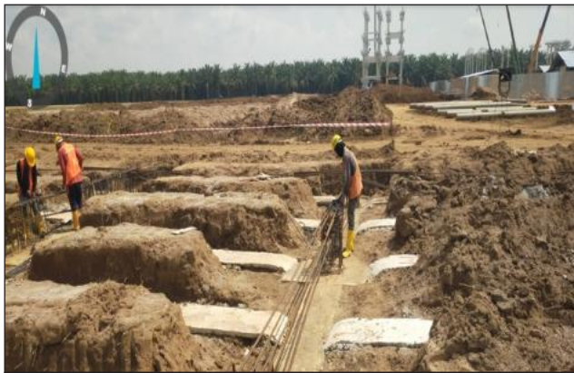
Installation of Rebar Reinforcement for Foundation
