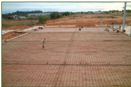
Slab Bor Laying
