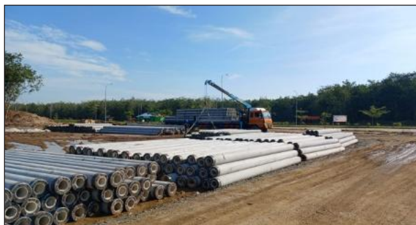
TMC Unloading Material At Laydown
