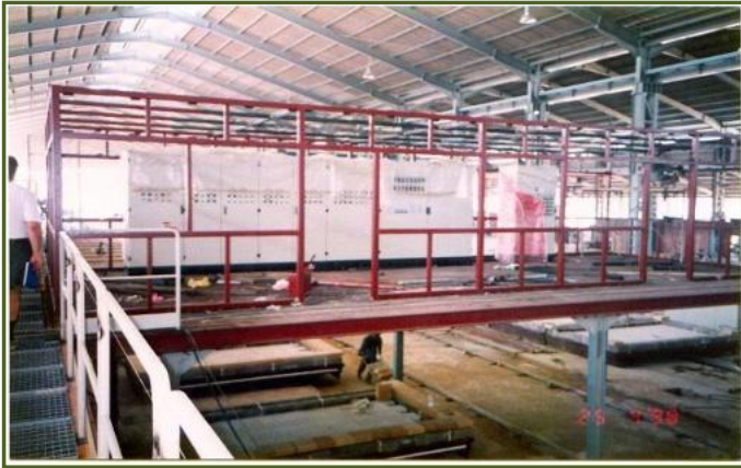
Electrical & Mechanical Control Room
