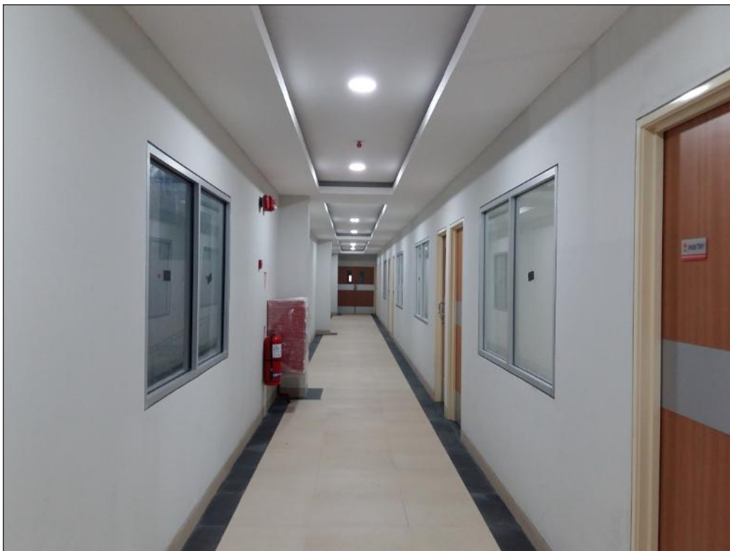
Installation Office of Window and Doors
