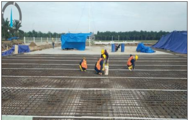
Cleaning Rebar Cuttings
