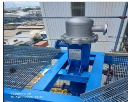
Install Equipment 3E-205 (Condensor) (Elevation +19.000)
