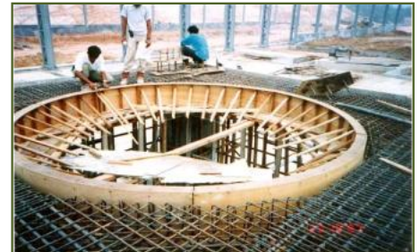
Construction of Pan Mill
