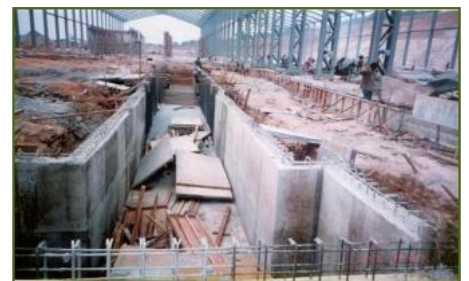
Construction of Trenches for Convenyor Belts
