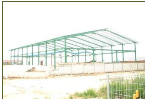
View Steel Structure
