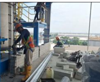
Install Brickwall Marshalling Room
