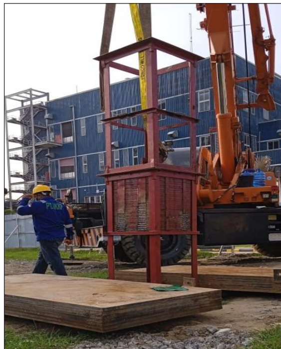
PDA Test Using Tower Method
