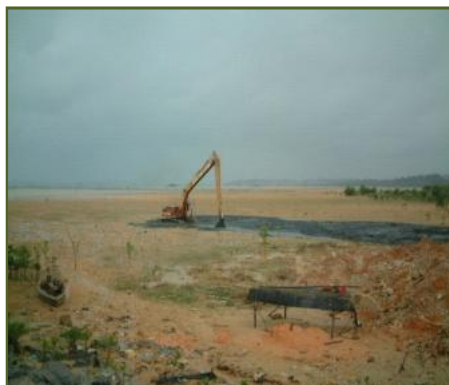
Removing Mud & Soft Soil
