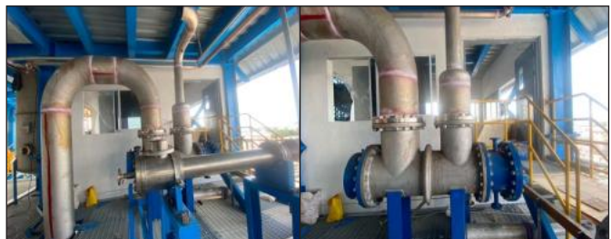
Completed Marshalling Room
