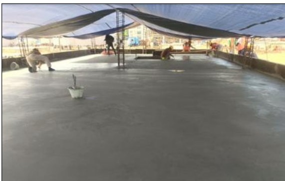
Concrete Floor Finishing Process Area Substation
