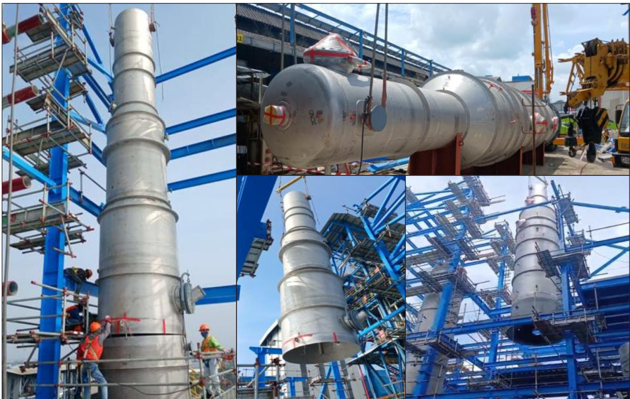
Install Equipment 3C-303 (Fatty Acid Receiver) (Elevation +6.000)
