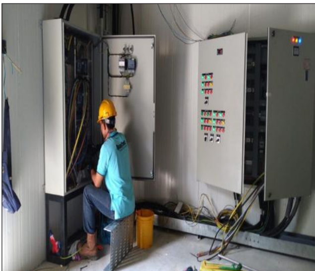
Termination of Electrical Panel
