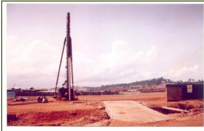
First Piling Works
