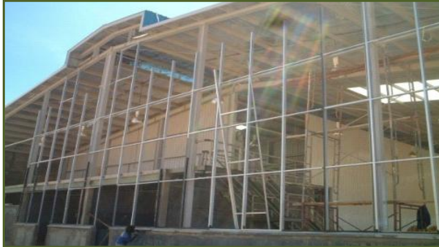
Installation of Curtain Wall
