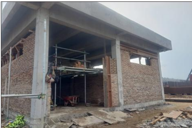
Brick Wall Installation at Substation Area
