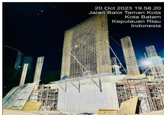
Reinforcement Installation for Shearwall
