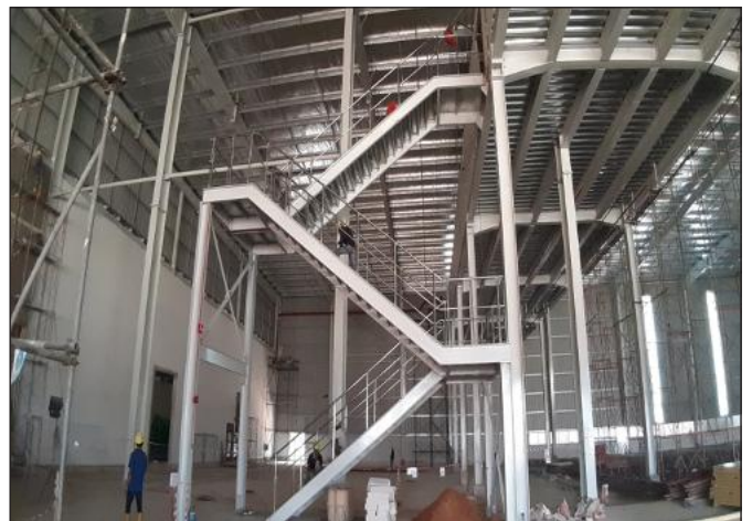
Erection of Internal Staircase for Mezzanine
