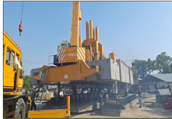
Unloading HSPD on Site
