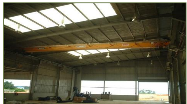
Overhead Crane Installation
