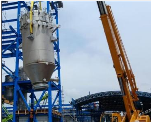
Install Equipment 3F-202A (Catalyst Filter) (Elevation 13.000)
