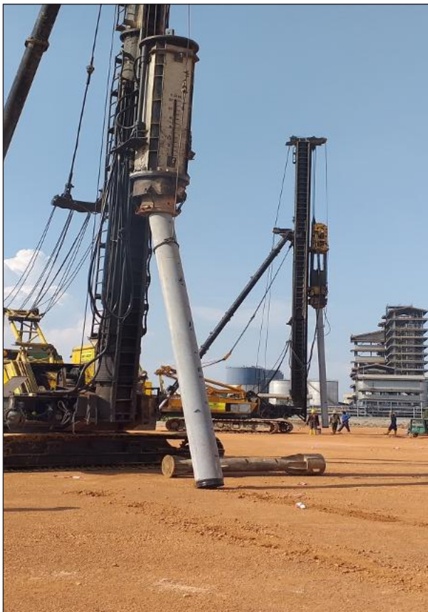
Lifting of Pile
