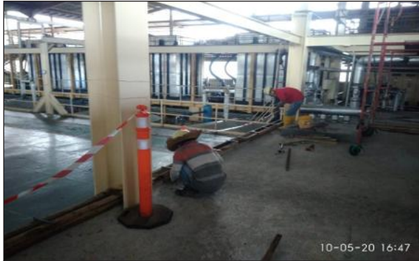
Formwork Installation for Kerb CPO
