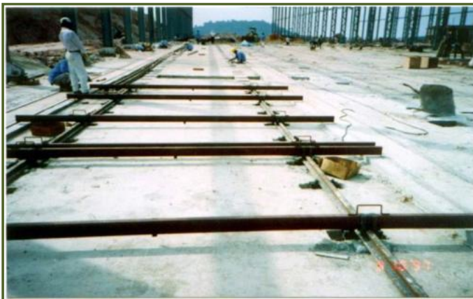
Installation of Rail Tracks for Kiln Car
