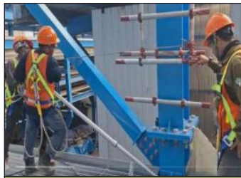
Torque Tightening Bolt
