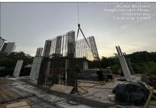
Reinforcement Installation for Shearwall
