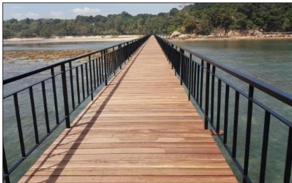
Installation of Timber Planks
