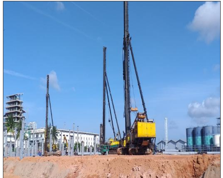
Driven of Pile
