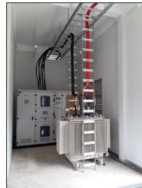
Installation of Transformer & LVMDP
