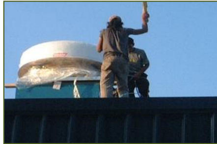
1500mm dia. Motonsed Extra Fan
