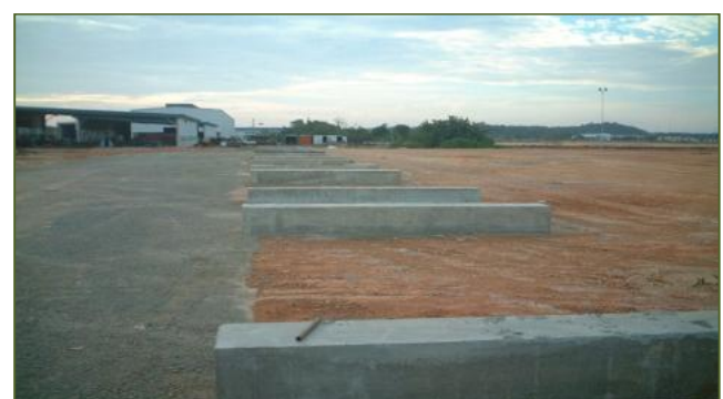
Concrete Sleeper for Steel Pipe
