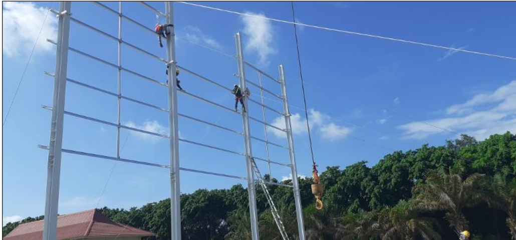
Erection of Wall Purlin
