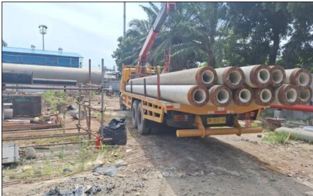
Loading & Unloading Material Pile
