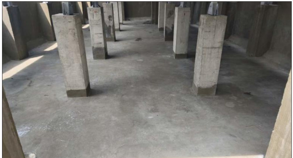
Completed Concrete Works
