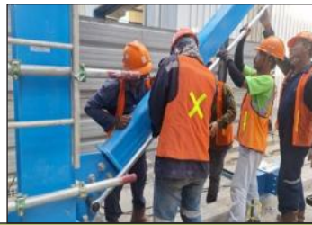
Torque Tightening Bolt
