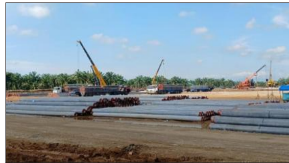
Laydown Area For Temporary Material
