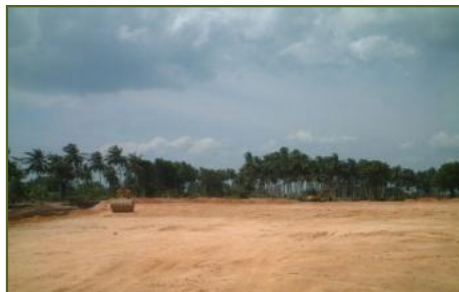
Landfill & Compaction As at 20 August 2003
