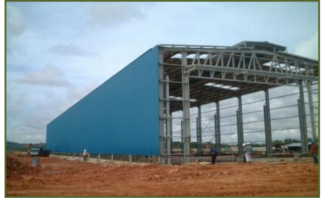
Installation of Metal Wall Cladding & Roofing
