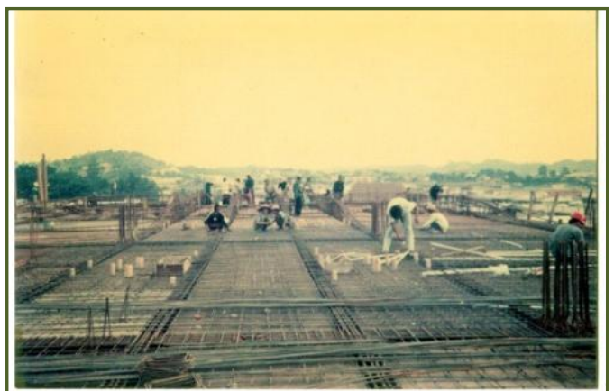
Slab for Reinforcement for Level 4
