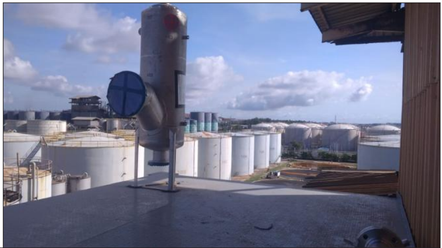
Installation of Vacuum Production
