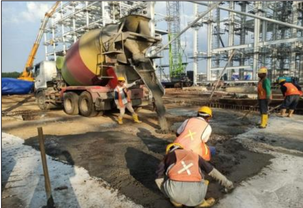
Execution Of Lean Concrete Work At Apron Area
