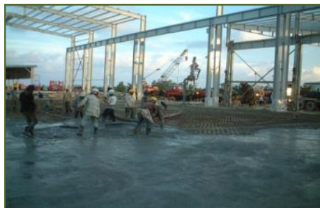
Slab Concreting
