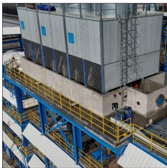
Completed Cooling Tower Installation
