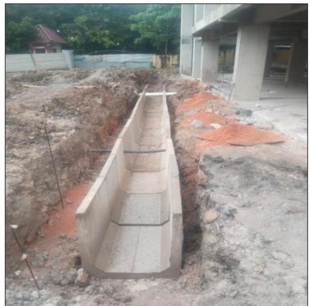
Perimeter Drain Works
