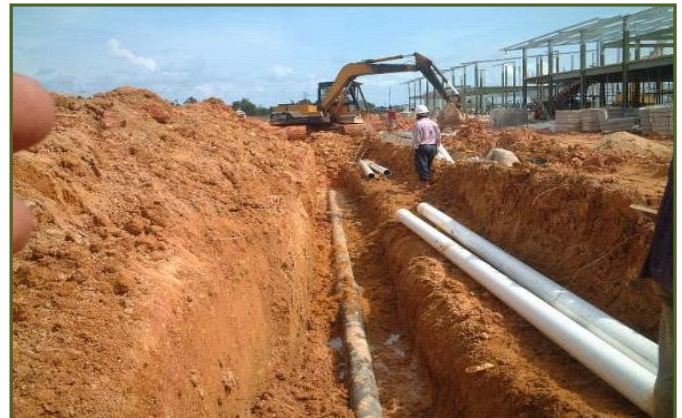
Installation of Ductile Iron Pipe for Main Water Line & PLN Conduit
