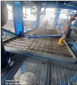
Install Rebar Marshalling Room
