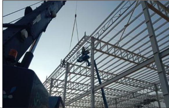
Steel roof truss and purlin installation in progress
