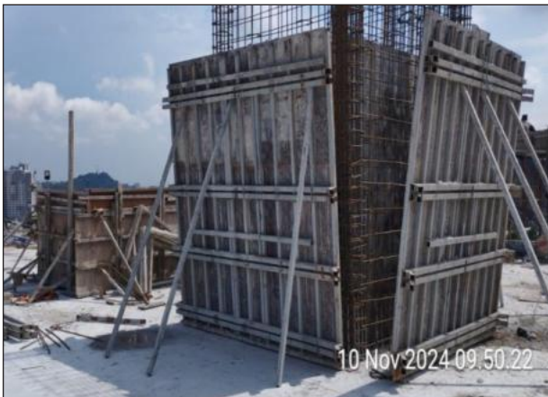
Reinforcement Installation for Roof Shearwall
