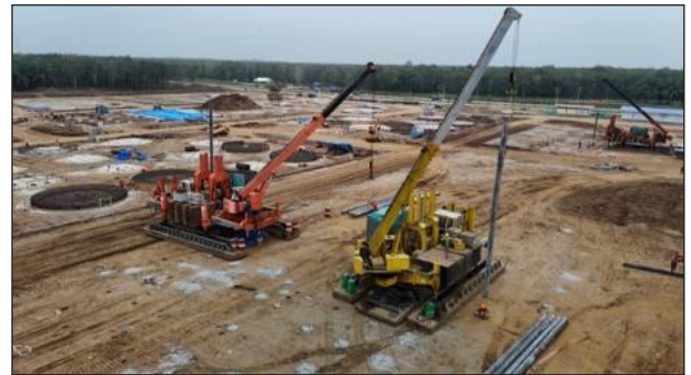
HSPD View Of Piling Work In Each Area
