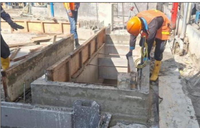
Dismantle Formwork Bundwall Fat Trap
