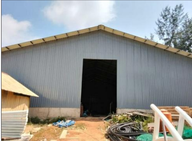
Subject : Steel Workshop Location : Kabil, Batam Island
