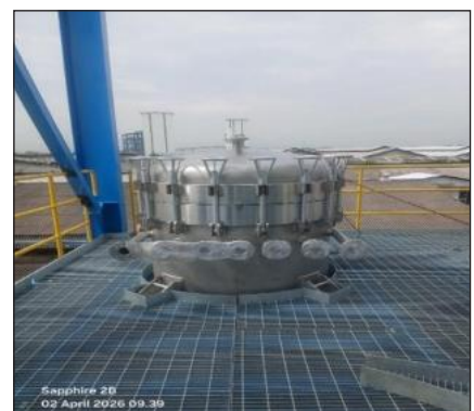
Install Equipment 3F - 202A (Catalyst Filter)(Elevation +13.000)
