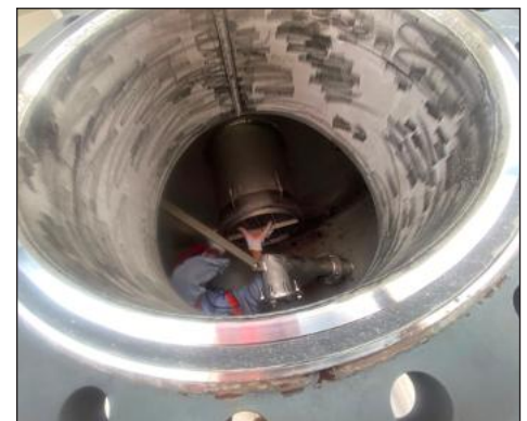
Collector Installed
