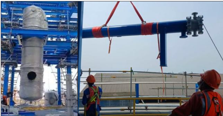
Install Equipment 3C-754 (Scrubber) (Elevation +18.000)
