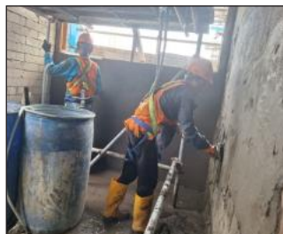
Internal Wall Plastering In The Marshalling Room
