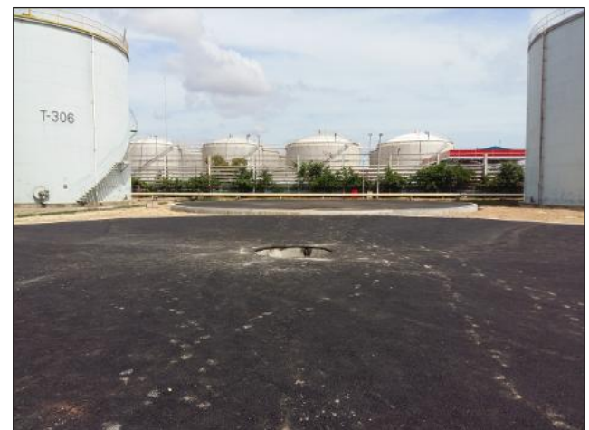
Asphal Layer for Tank 7500MT
