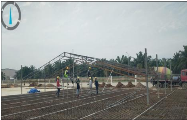
Installation of Warehouse Panel Roof Frame
