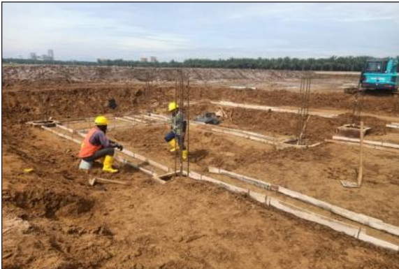
Install Formwork LC Area Substation
