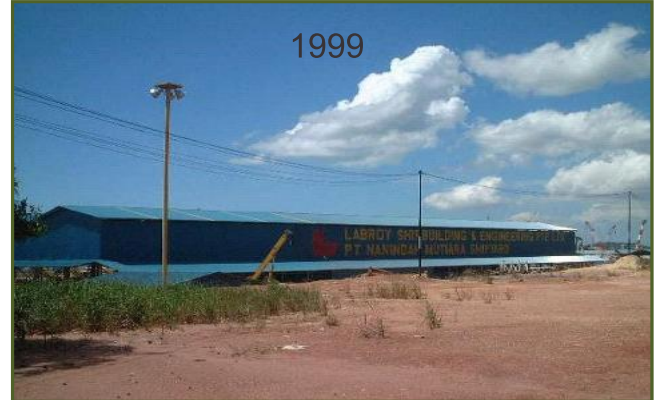
PT. NANINDAH MUTIARA SHIPYARD (Factory & Office Building)
