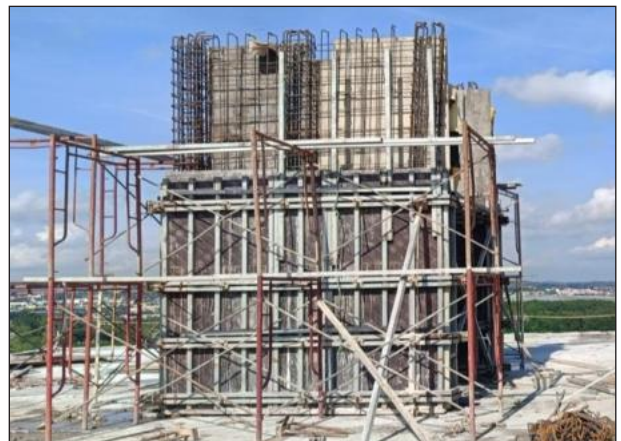
Reinforcement Installation for Roof Shearwall
