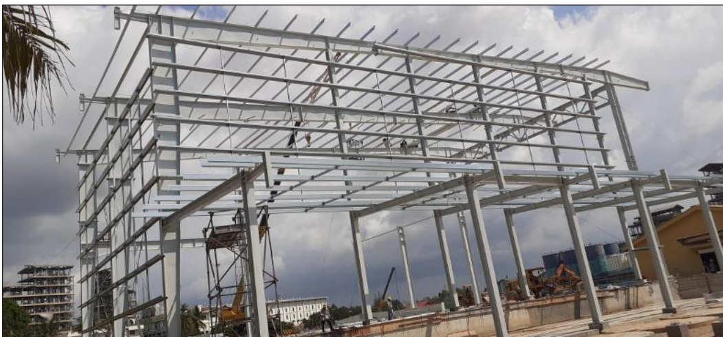
Erection of Roof Purlin
