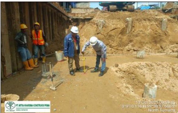
Inspection and Measurement of Ground Level After Compaction
