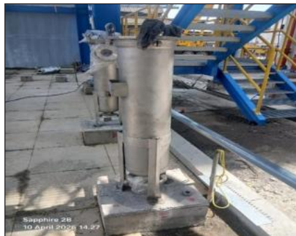
Install Equipment 3F-201B (Feed Filter)(Elevation. 0.000)
