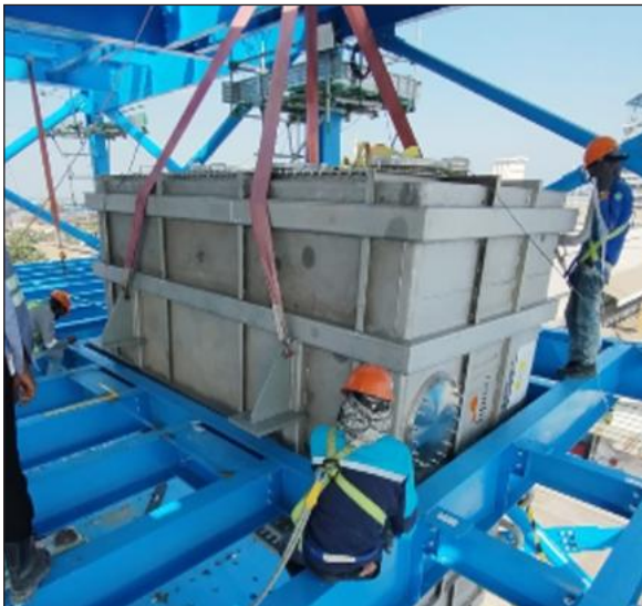
Tank Lifting Setting Centerline D-661
