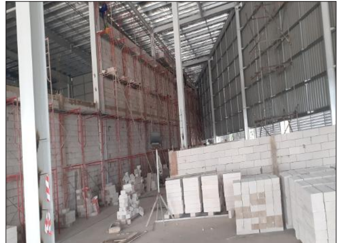
Installation of 12 Meter Brickwall Hight at Finish Good Warehouse Area
