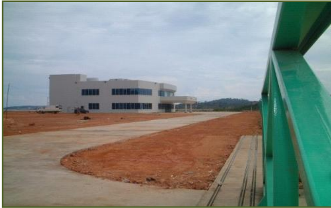
Concrete Road/Pavement to Main Office
