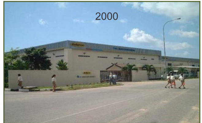
PT. RUBYCON INDONESIA (Factory & Office Building)
