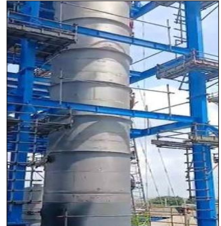
Install Equipment 3C-754 (Srcubber) (Elevation +18.000)
