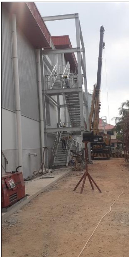
Erection of Staircase for Condensor Area
