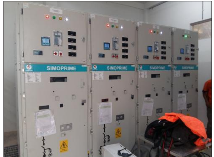
Installation of LVMDP 2500 Kva x 2
