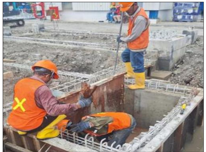
Dismantle Formwork Bundwall Fat Trap
