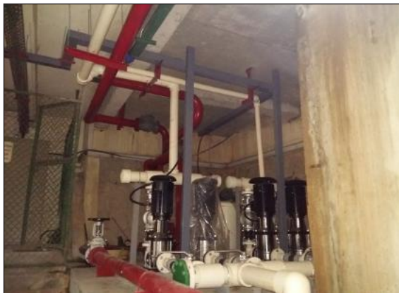
Installation of Pump
