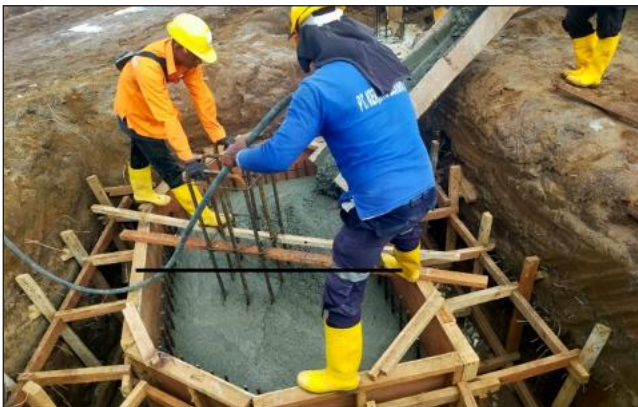
Foundation Concrete Casting Process
