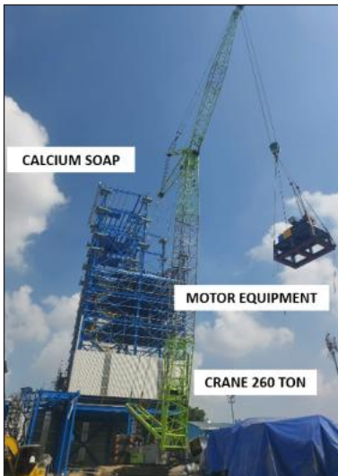
LIFTING OF MOTOR EQUIPMENT
