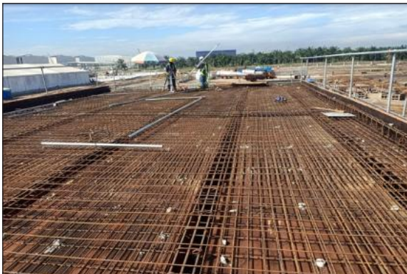
Rebar Panel Installation Area Substation
