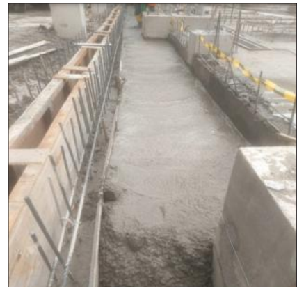
Rebar Installation and Foundation Concrete Casting with Proper Compaction
