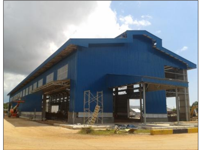
Installation of Roof & Wall Clading
