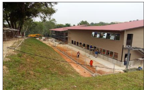
Cladding & Roofing Installation
