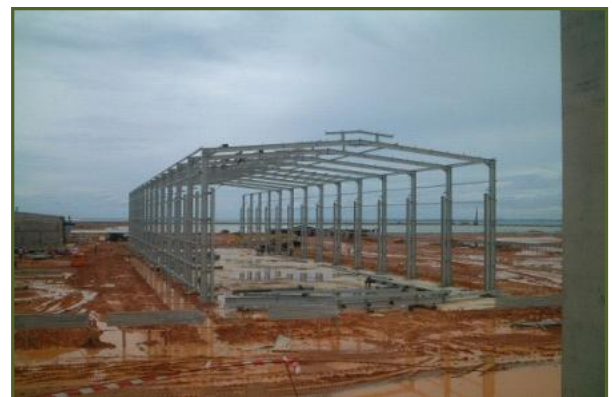
Steel Structure Frames of Fabrication Shop
