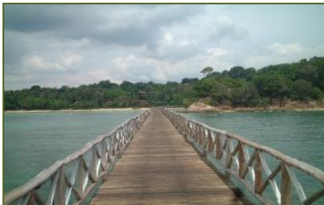
Timber Floor & Railing
