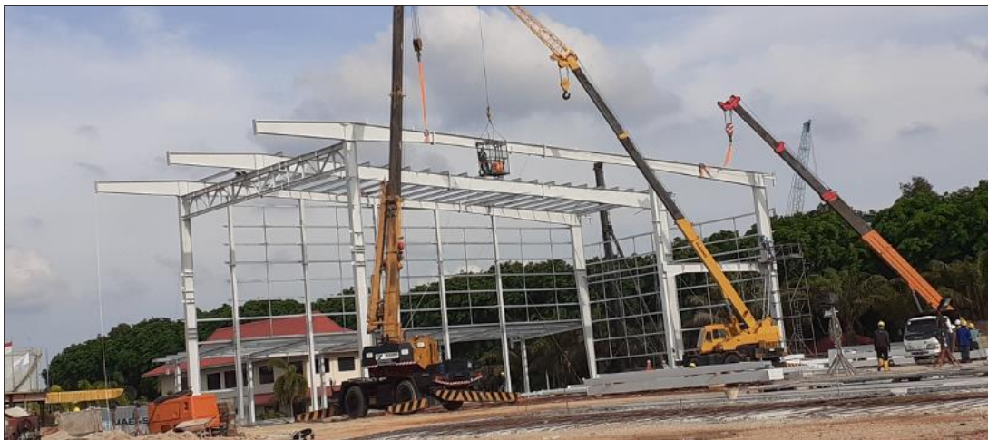
Erection of Column
