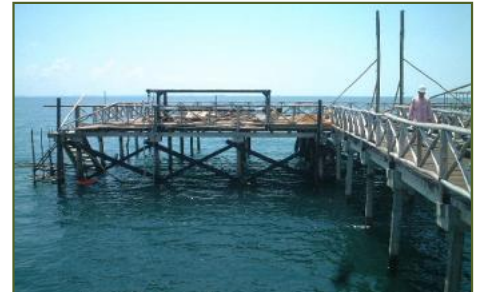
Timber Bracing
