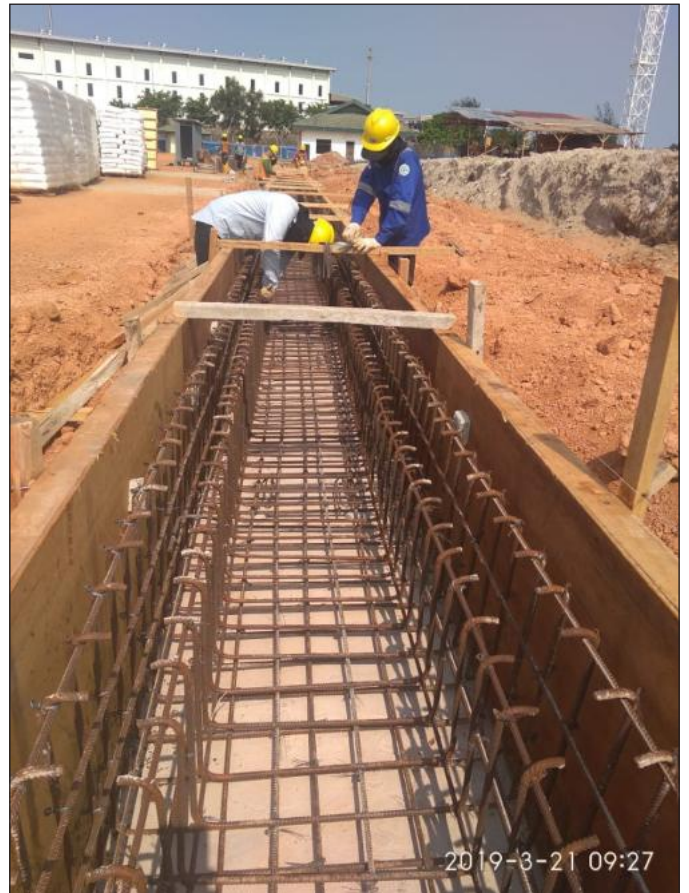
Reinforcement Installation for Drain
