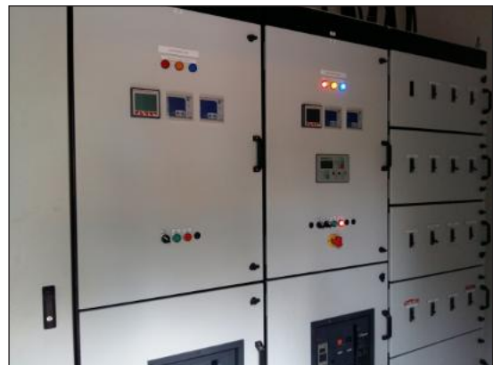
Installation of LVMDP
