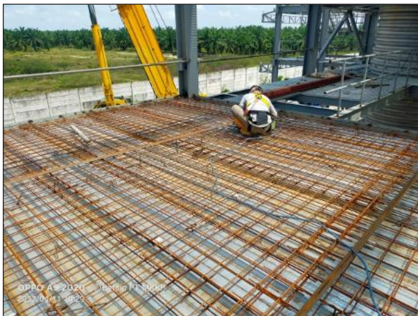
Bondex Concrete Floor at Level +5.00
