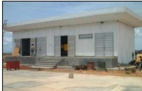
Front View of Power House
