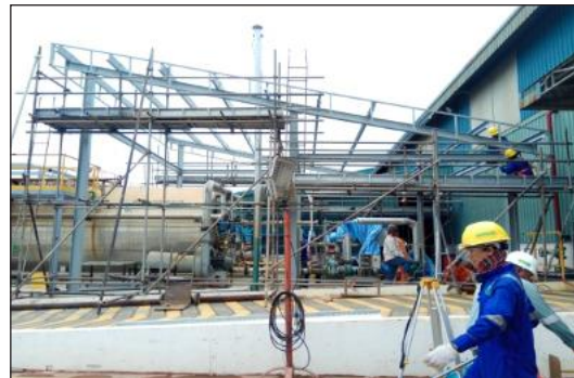
Erection of Steel Structure
