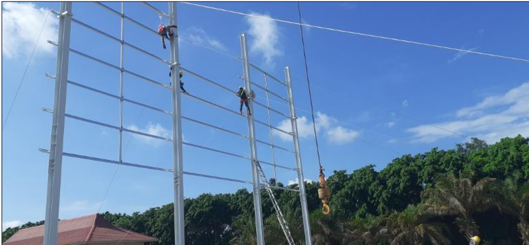
Erection of Wall Purlin
