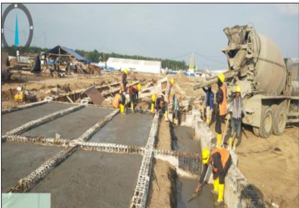
Execution Of Lean Concrete Work At Apron Area
