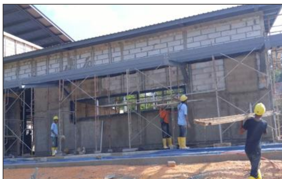
External Wall Installation
