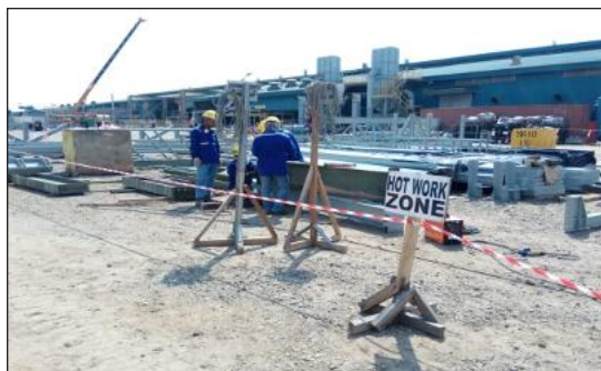
Fabrication of Steel Structure
