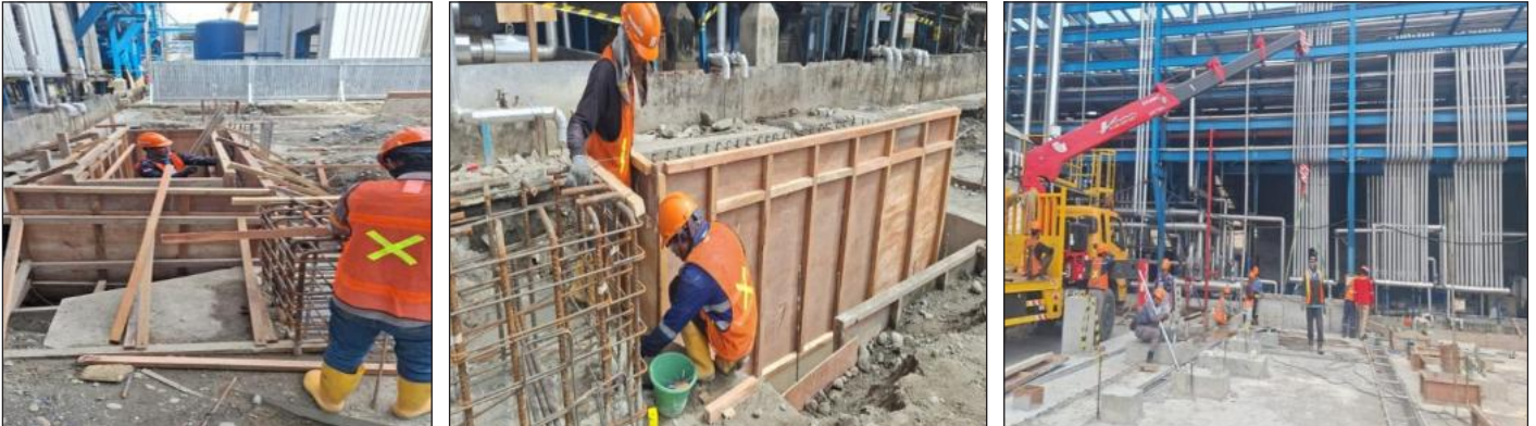
Install Formwork dan Install Lining Fat Trap
