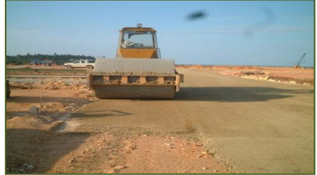
250mm Thick Basecourse Pavement
