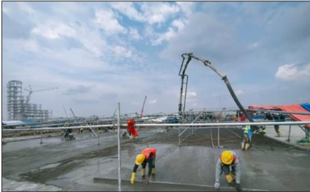
Concrete Casting Process
