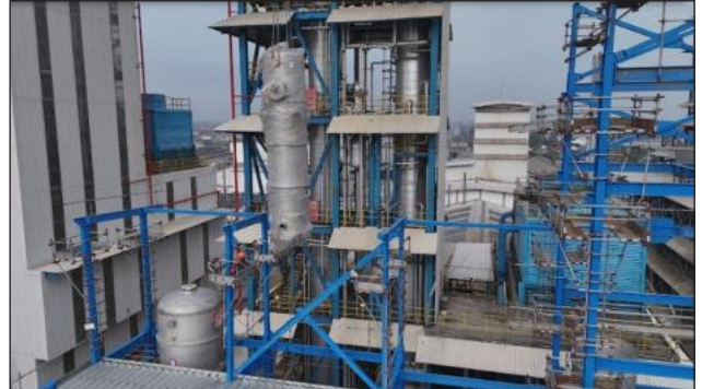
Install Equipment 3C-754 Using Crane 260 Ton (Elevation +18.000)
