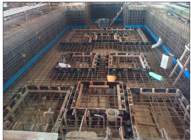
Reinforcement of Tilting Foundation Works
