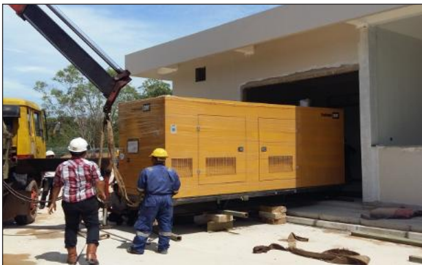
Installation of Generator
