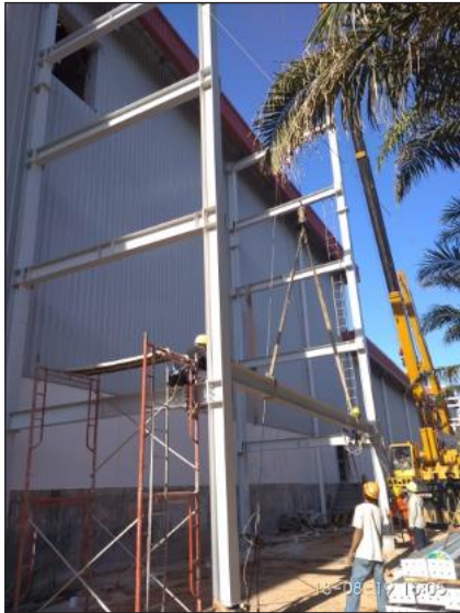
Erection of External Staircase for Mezzanine
