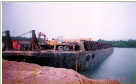
Heavy Equipments Arrived on Site
