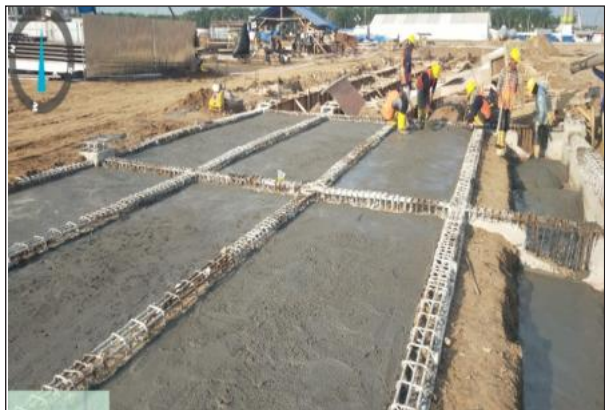
Execution Of Lean Concrete Work At Apron Area
