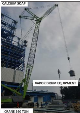
LIFTING OF VAPOR DRUM EQUIPMENT
