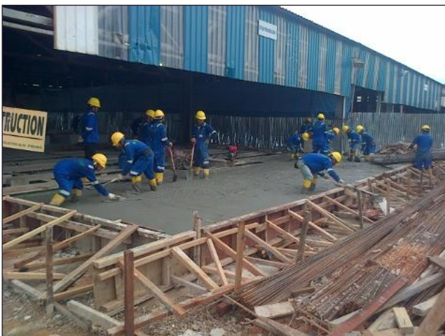
Concrete Slab Works
