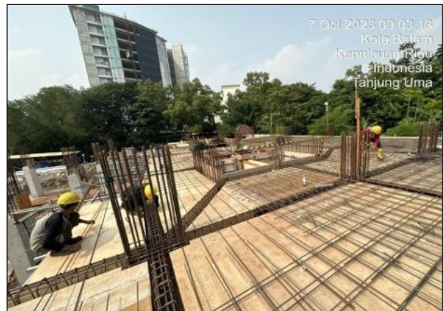
Reinforcement Installation for Slab Works
