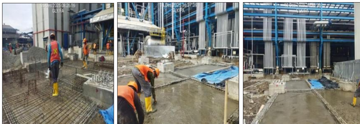
Reinforcement and Concrete Pouring Work for GLY/FA Area Slab
