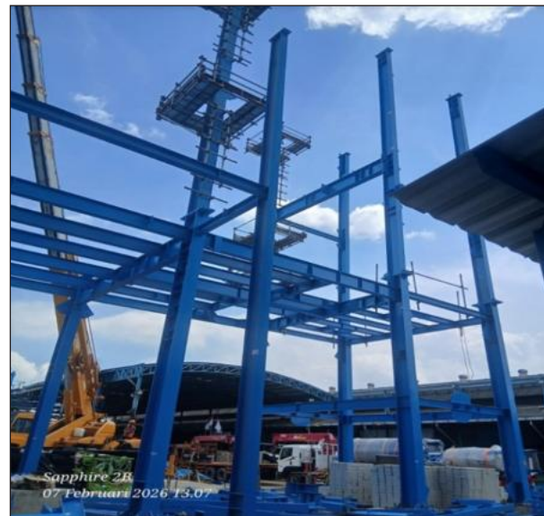
Erection Column Oil Hydrogenation Plant
