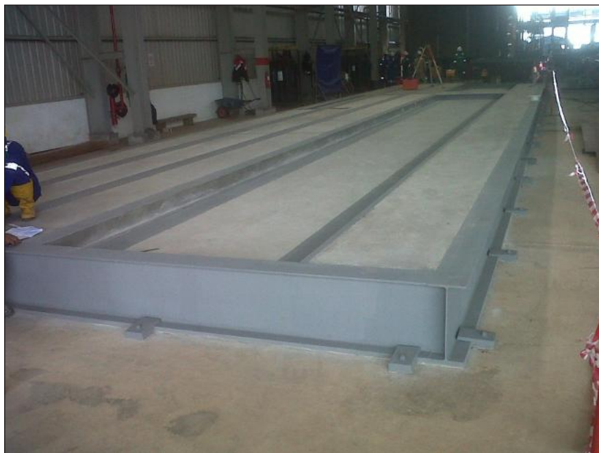
Concrete Foundation Work
