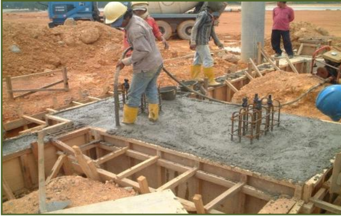
Pile Cap Concreting
