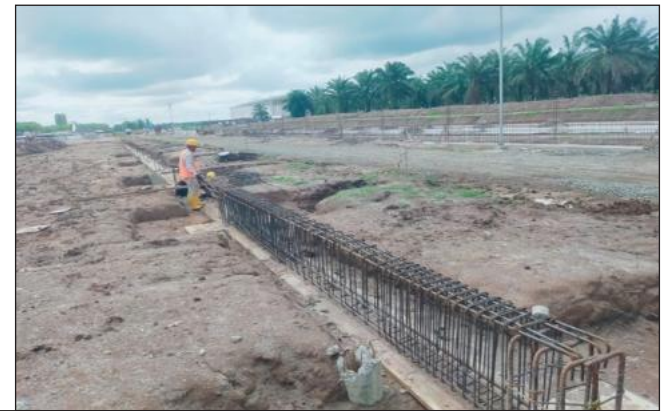
Installation of Rebar Reinforcement for Foundation
