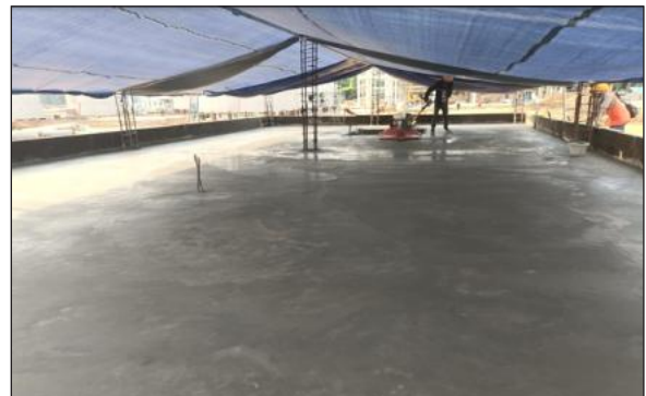
Concrete Floor Finishing Process Area Substation
