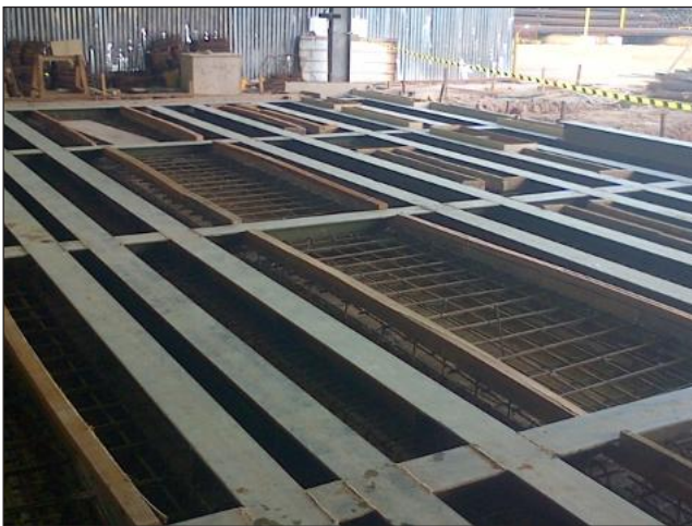
Steel Structure Works
