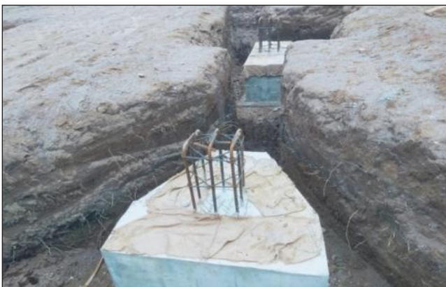
Foundation Structure Completed Casting
