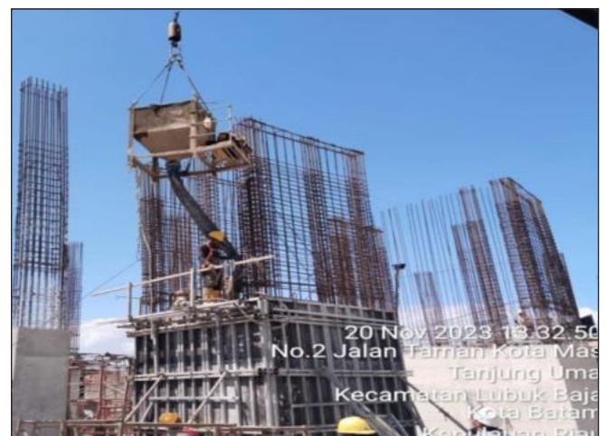
Concreting Works
