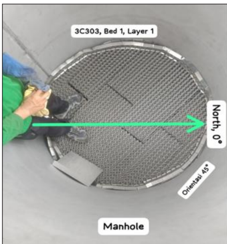
Support Grid Installed
