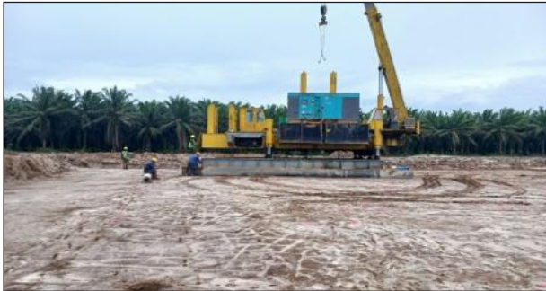
HSPD On Position For Piling Work
