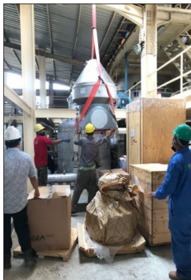
Installation of Separator
