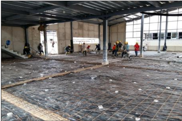
Reinforcement Works
