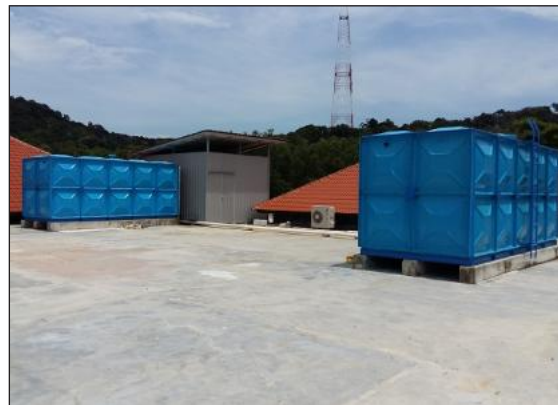
Installation of Water Tank
