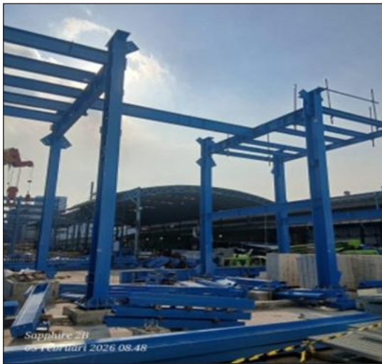
Erection Beam Oil Hydrogenation Plant
