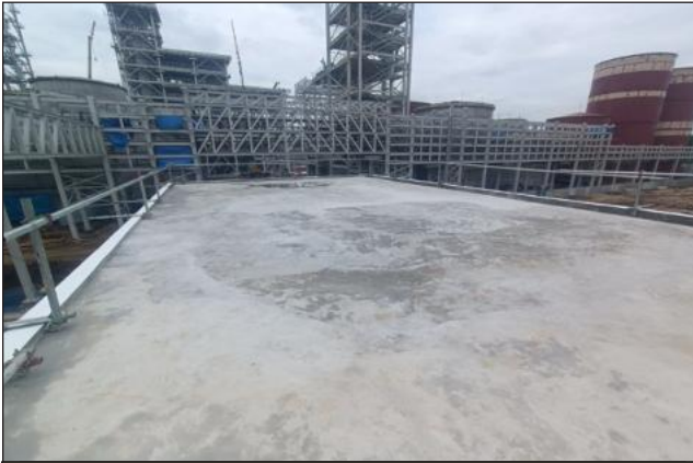
Roof Screeding Works at Substation
