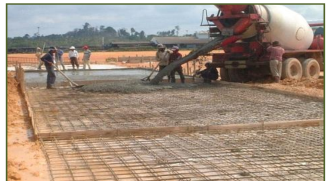
Concrete Pavement
