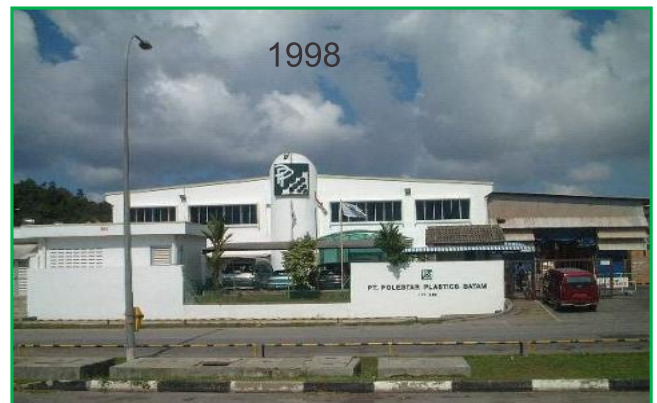
PT. POLESTAR PLASTIC BATAM (Steel Structure & Building Works)
