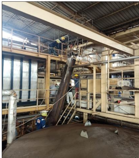
Erection of Steel Beam
