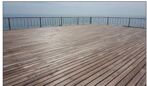
Installation of Timber Planks
