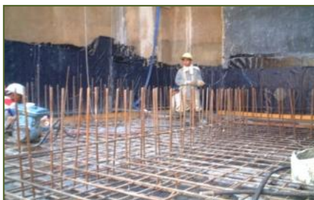
Waterproofing Membrane & Reinforcement for Reservoir Floor at 5.00 Dept
