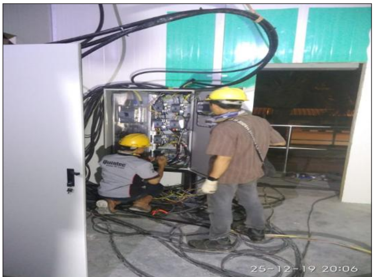
Termination of Electrical Panel
