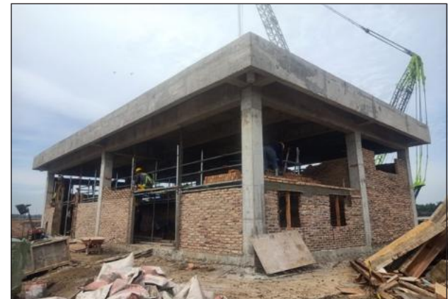
Brick Wall Installation at Substation Area
