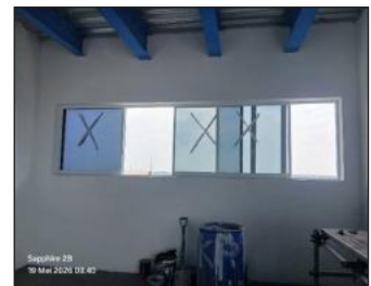
Installation Windows Marshalling Room
