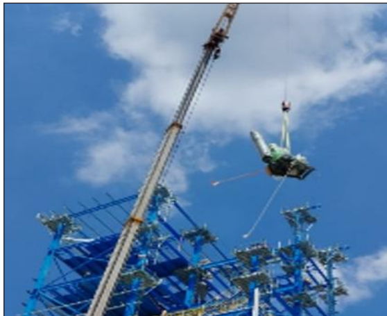
Pump Lifting
