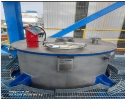
Install Equipment 3D - 201 (Deareator Heater) (Elevation +7.000)
