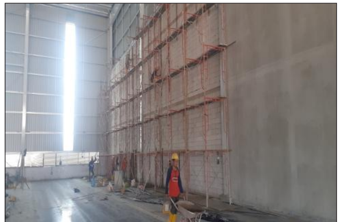
Installation of 12 Meter Brickwall Hight at Raw Material Warehouse Area
