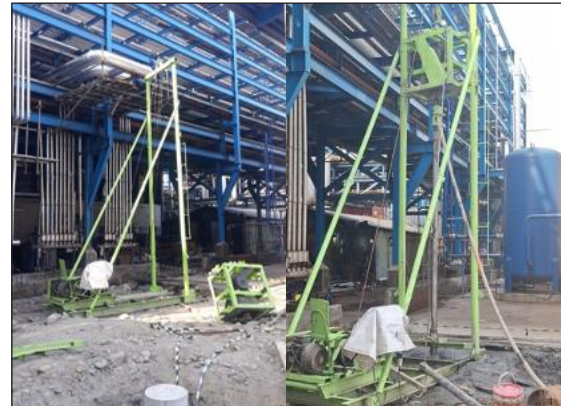
Assembling Equipment Bored Pile
