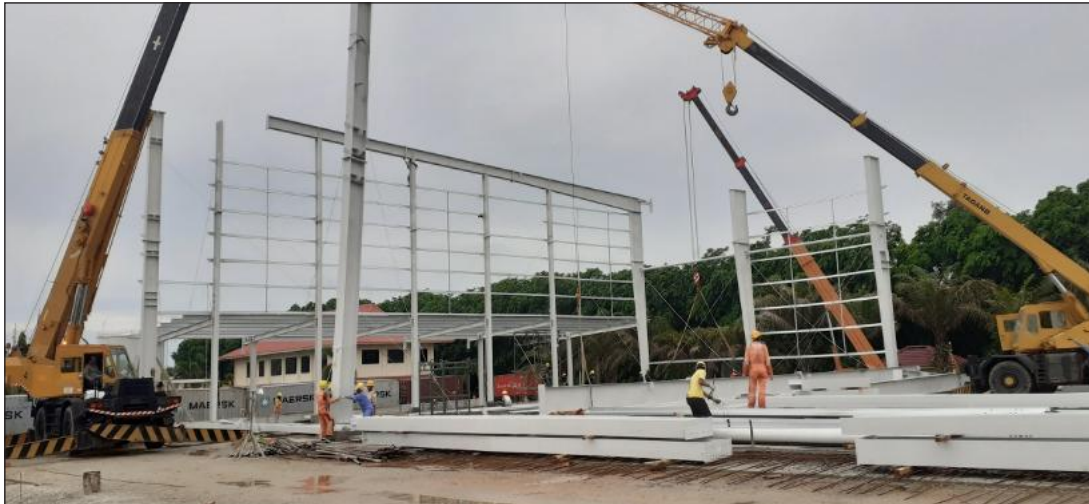
Erection of Column
