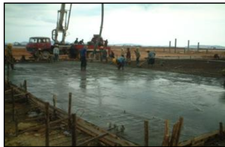
Floor Slab Concreting
