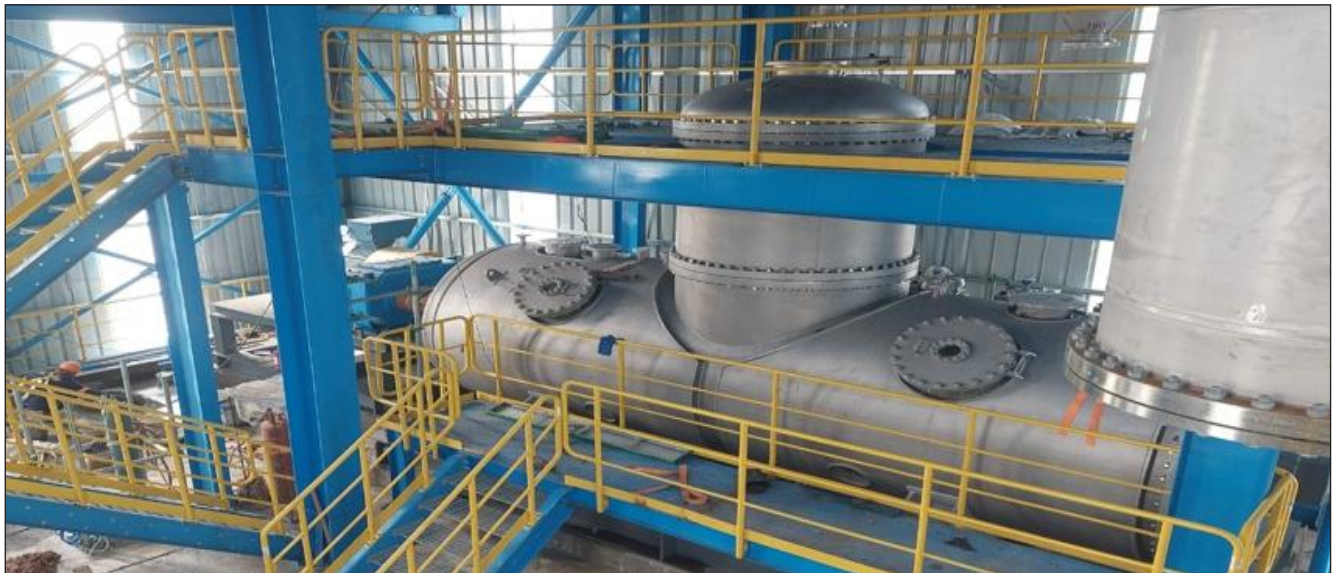
ALL EQUIPMENT AND PLATFORM ALREADY COMPLETED
