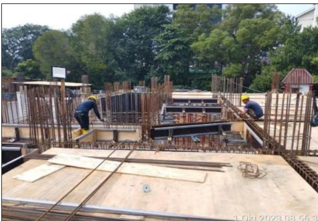
Reinforcement Installation for Slab Works
