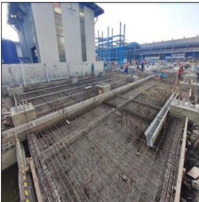
Rebar Installation and Foundation Concrete Casting with Proper Compaction
