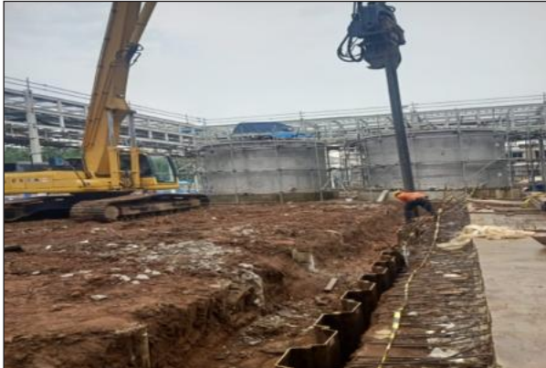
Sheet Pile WTP Area
