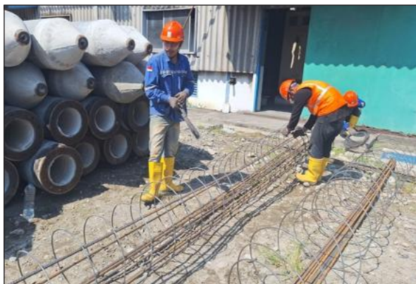
Rebar Bored Pile Fabrication
