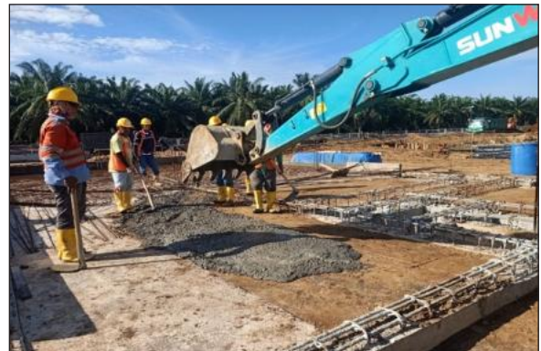
Lean Concrete Work Area Substation
