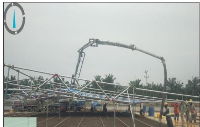
Warehouse Panel Floor Casting Process
