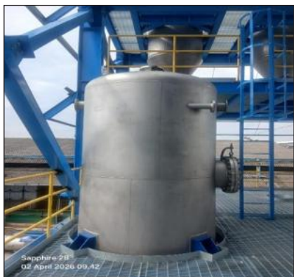
Install Equipment 3D - 203 (Filtered Product Receiver) (Elevation +7.000)
