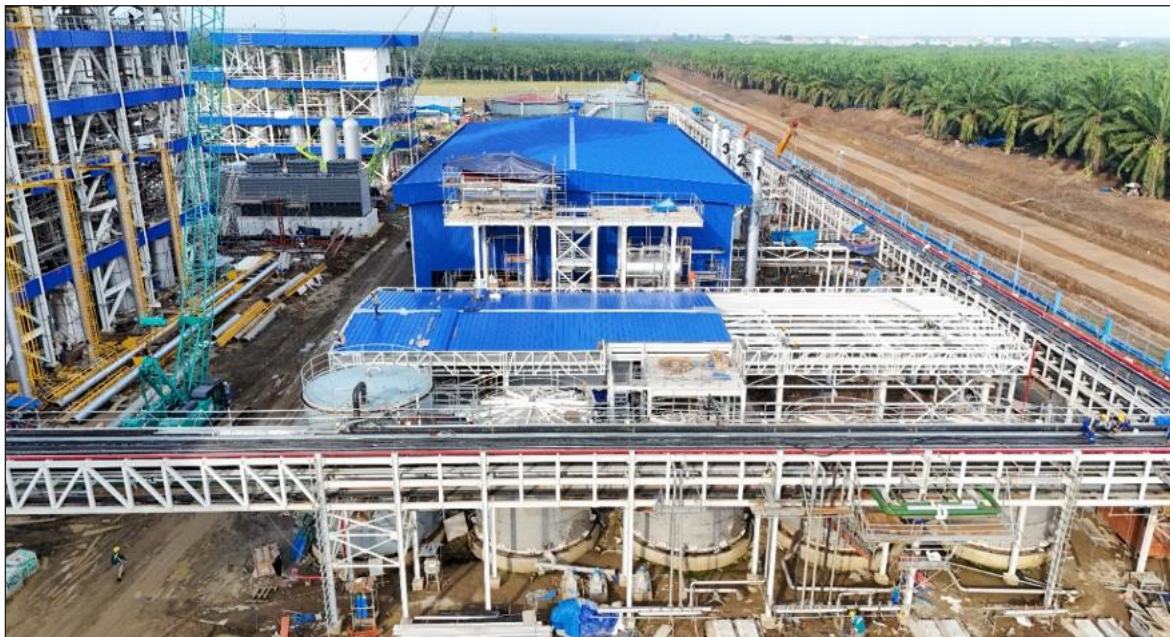
Front view of the boiler house
