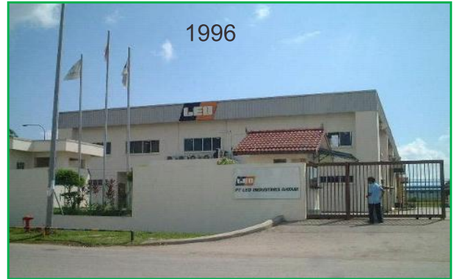
PT. LEO SAKATA (Steel Structure & Office Renovation)
