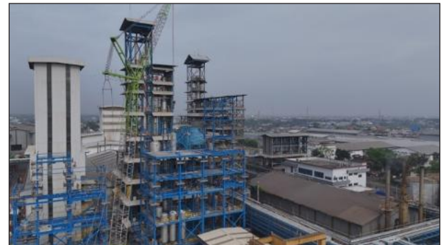
Install Equipment 3C-754 Using Crane 260 Ton (Elevation +18.000)
