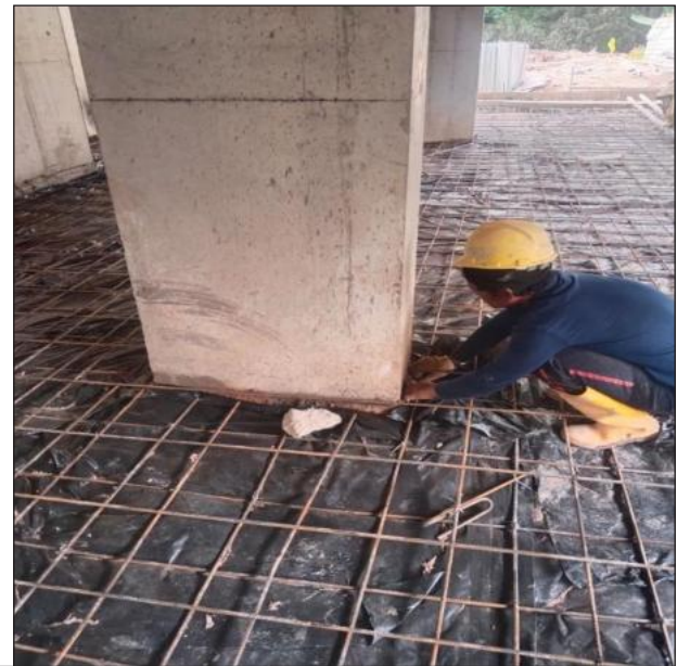
Reinforcement Installation for Slab Works
