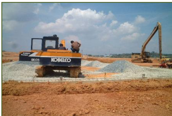
Base Course Laying
