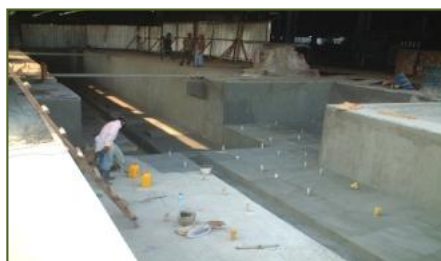
View of Machine Foundation
