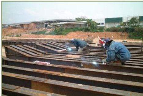
Fabrication of Steel Structure
