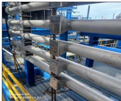
Install Equipment 3E-203 (Heat Recovery Exchanger)(Elevation +7.000)
