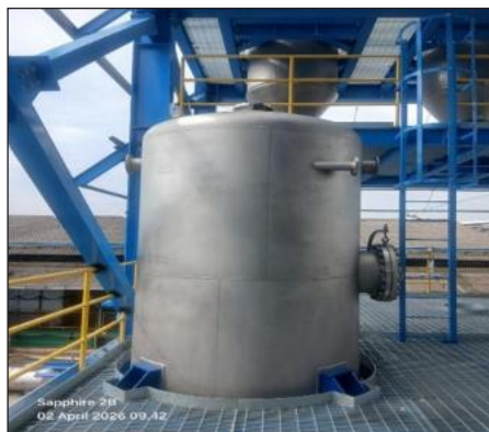
Install Equipment 3D - 203 (Filtered Product Receiver) (Elevation +7.000)
