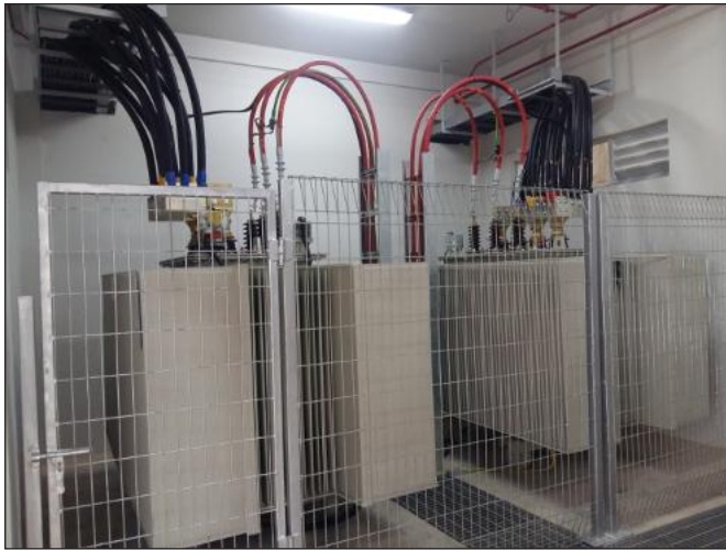
Installation of Transformer 2500 Kva x 2
