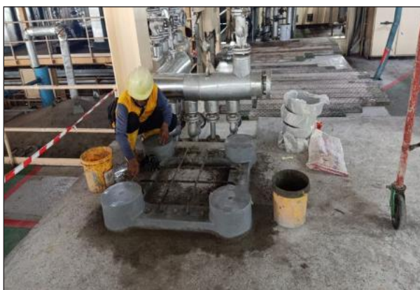
Grouting of Foundation Equipment
