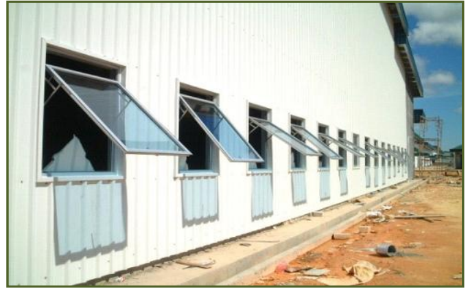
Installation of Aluminium Windows & Metal Trims
