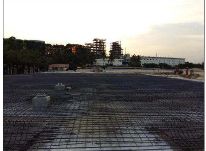
Reinforcement Installation for Slab
