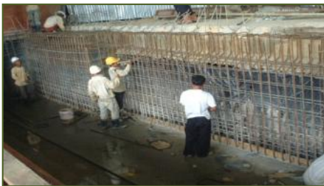
Waterproofing Membrane & Reinforcement for Machine Foundation Wall
