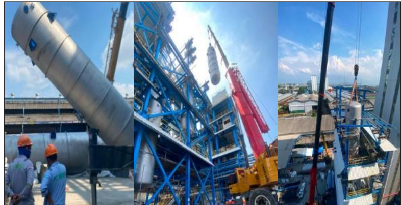
Install Equipment 3C-201 (Deareator Heater) (Elevation +19.000)
