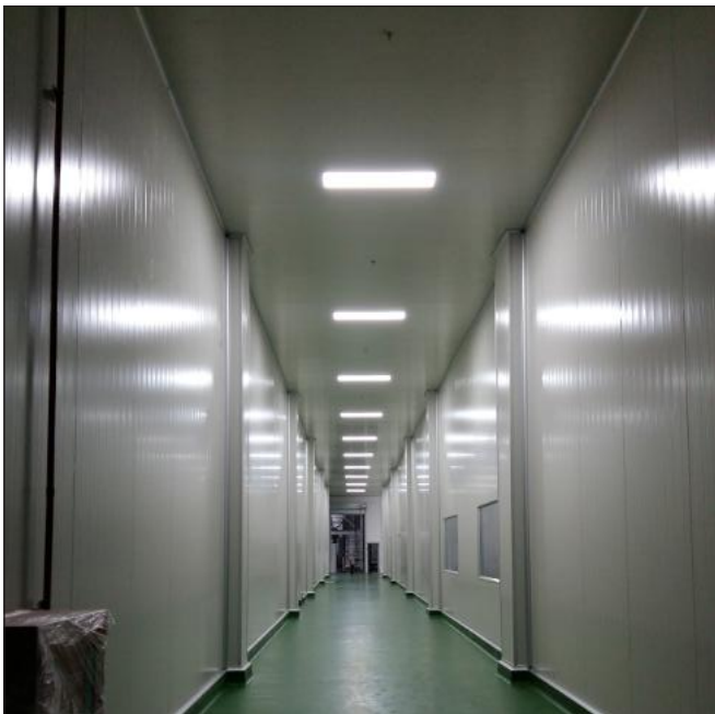
PU Flooring Works at Filling Lines Area & Coridor
