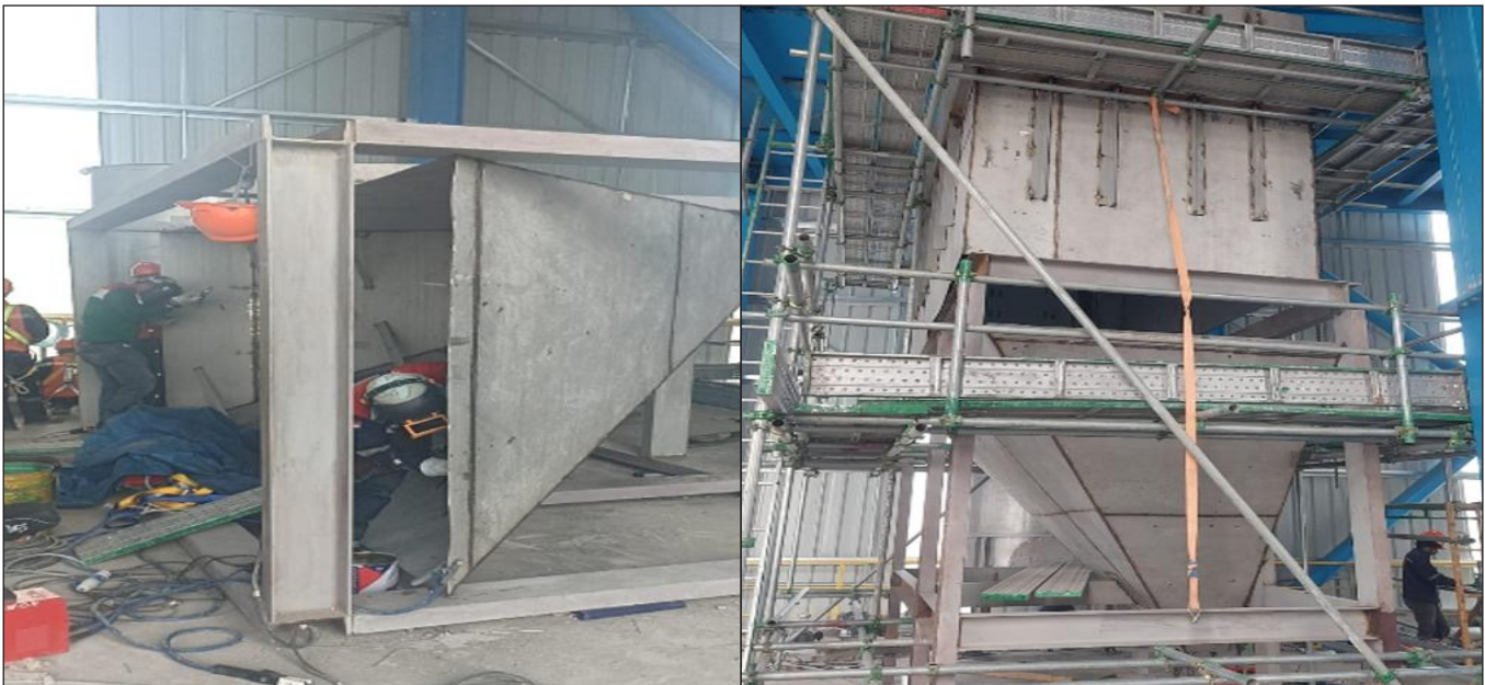
Fit Up and Welding Plate
