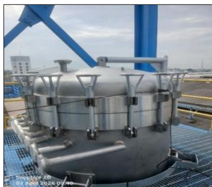
Install Equipment 3F - 202A (Catalyst Filter)(Elevation +13.000)
