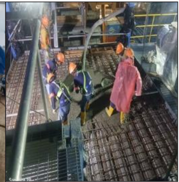
Pouring Concrete Slab Marshalling Room
