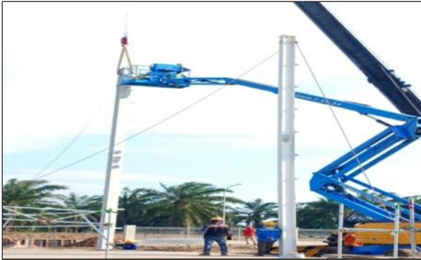
Column Erection at Warehouse
